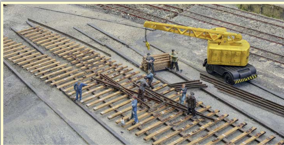
A track formation is being laid out in the yard. The way the foreman is pointing the finger it looks as though the sleeper numbering may have gone awry!
