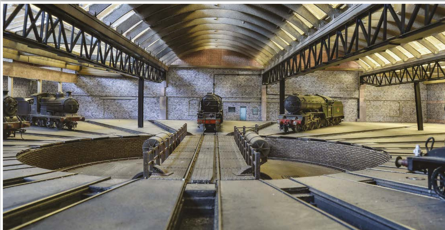
We had fun producing this one. The roof was removed, camera placed, and set on a 10-second timer for the roof to be replaced. The roof girders were profiled from drawings from the planning application to convert the shed to the National Railway Museum, obtained from York City Council.
