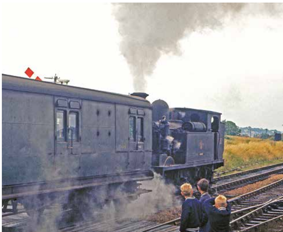
Departing Shanklin, bound for Ryde Pier Head, number 33 Bembridge is the subject of much interest from three young enthusiasts. The four compartment bogie brake third coupled next to the engine is S4149, once a SE&CR seven compartment brake composite "birdcage", but converted on transfer to the island to give more luggage space and meet the clearance requirements.
