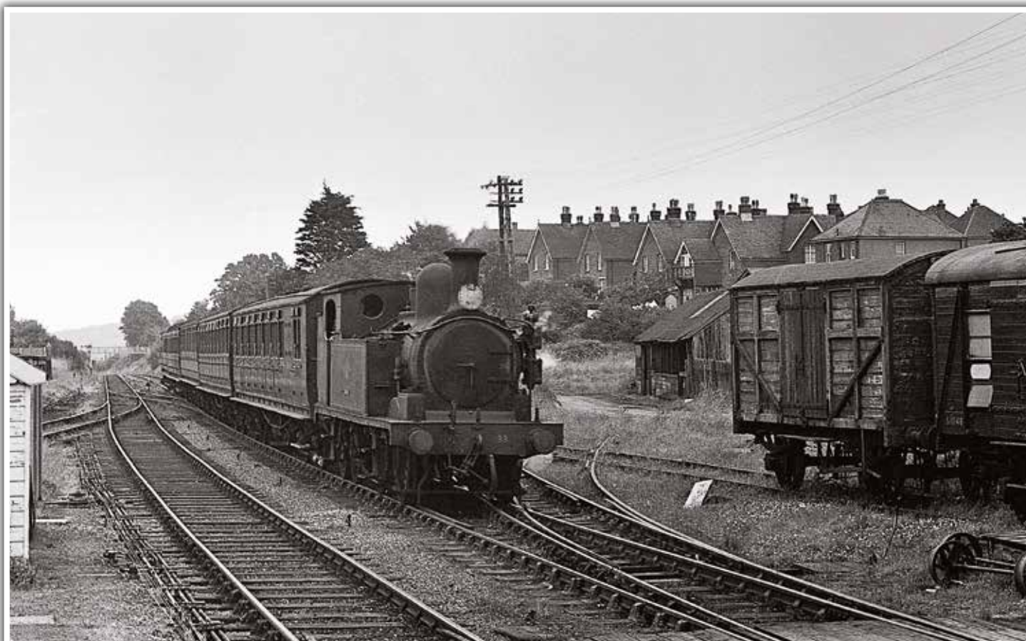
Having traversed the double-track section from Brading, No. 33, Bembridge arrives at Sandown, once the administrative headquarters of the Isle of Wight Railway Co. Note the goods-yard, rather over-grown, but the track formation with sidings cross-over is still visible. The covered vans, parked in one siding, once saw service as passenger advanced luggage vehicles. The van nearer the locomotive, a one-time 10-ton cattle wagon, originating from the LB&SCR, was converted to a standard van during 1935 after transfer to the island circa 1927-9.
