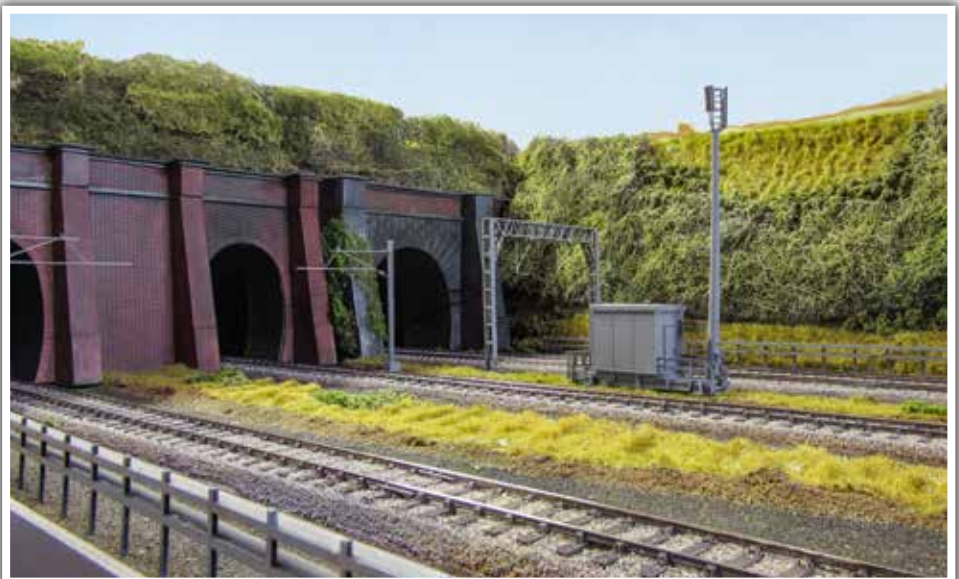
The low-down view of the southern portals of Northchurch Tunnel ahead of the wiring shows the proliferation of hardware around the modern railway, with electrical trunking on both sides of the line and raised equipment boxes associated with the communications mast.
