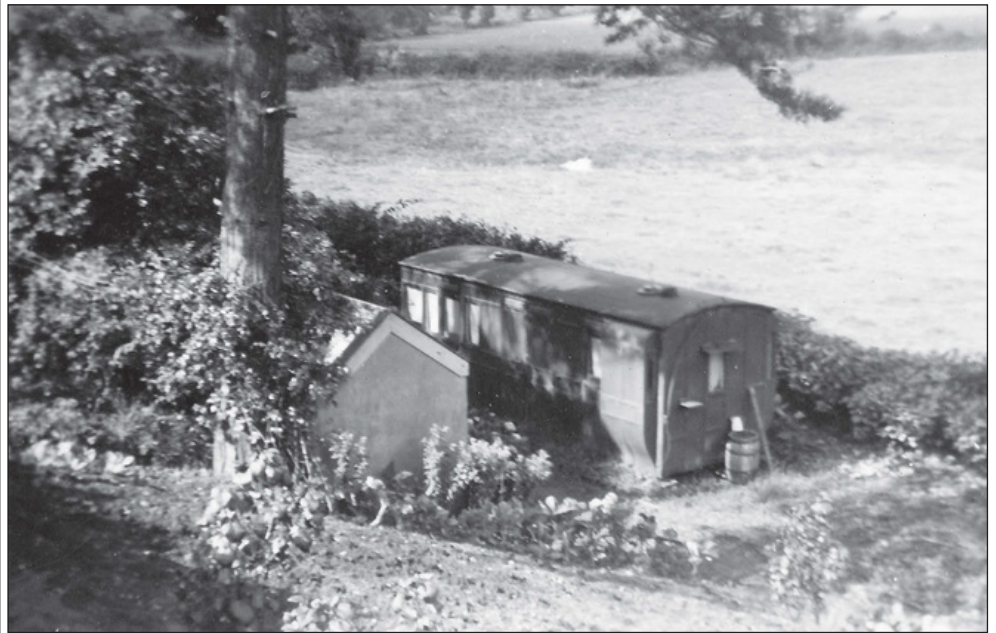
Above: Carriage no 1 had been turned into living accommodation at Snapper – sadly it fell victim to arson in the 1970s.
