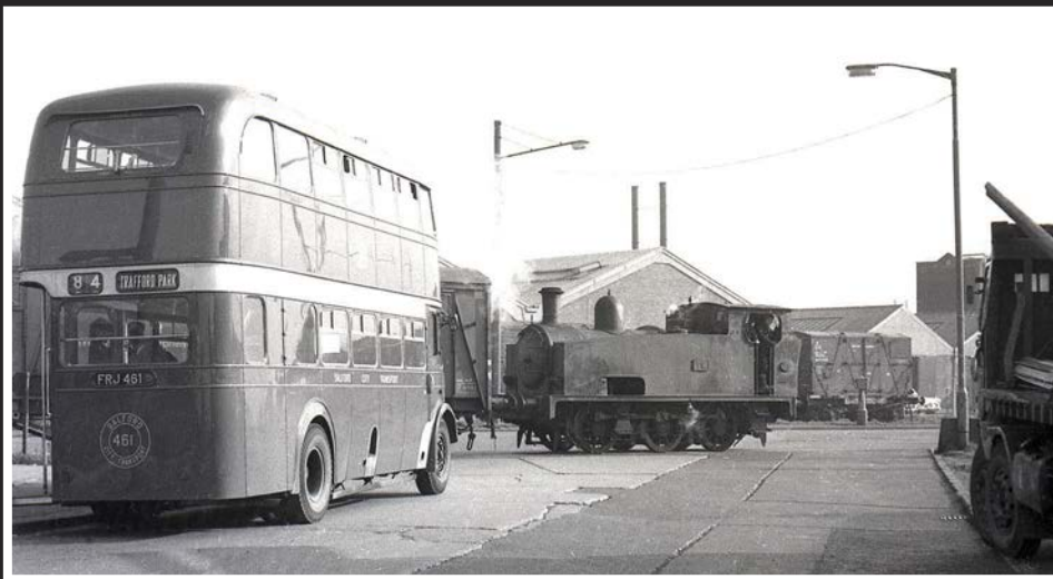
By 1965, only a handful of MSC Railway's once numerous fleet of steam locomotives were still in use, but these included No. 79, works No. HC1590 built 1927, which is pictured at the junction of Tenax Road and Trafford Park Road with a BR Ferry Van from CPC on October 19, 1965. The No. 84 bus route ran between Trafford Park and Davyhulme, while the 'Conflat A' loaded with a BD container, which can be seen standing on the line that ran along the north side of Trafford Park Road, was waiting to enter the nearby soap works of Thomas Hedley & Co.
