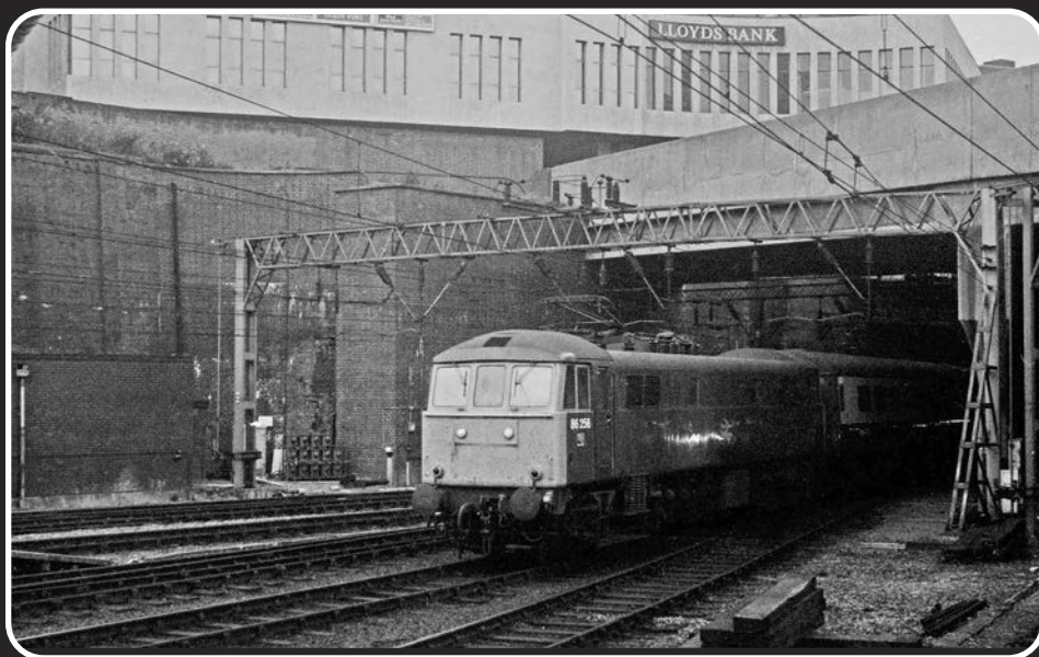
Access to Birmingham New Street Station from either the east or west is subterranean; not exactly through tunnels in the truest sense, but below buildings and streets. This image shows a Class 86 electric locomotive hauling a West Coast service into the eastern end of the station in 1978. Below the station platforms lies a warren of tunnels. Now redundant, they were once a means for long trains of mail trolleys, hauled by electric tractors, to transfer Royal Mail between the station and the city's vast sorting facility.
