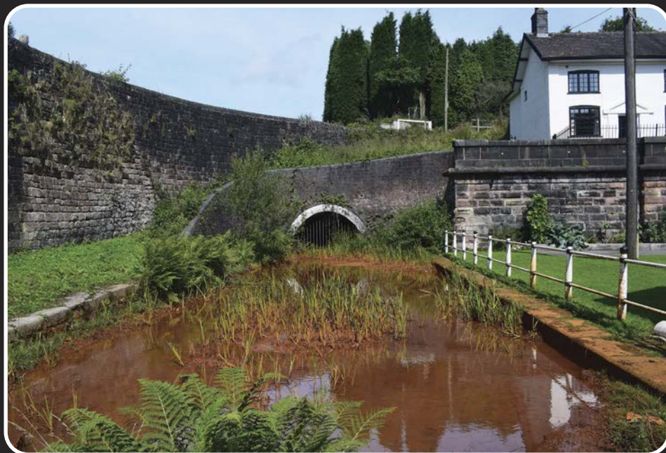
The northern portal to the first canal tunnel to be driven through Harecastle Hill; opened 1777, a second bore was cut in 1827 to handle the high amount of traffic. The original tunnel had to be closed in 1914 due to a partial collapse, possibly caused by vibration created from trains passing through the neighbouring railway tunnel. Nearby ironstone workings are responsible for the colour of the water. The portal to the surviving tunnel is to the right of this image.
