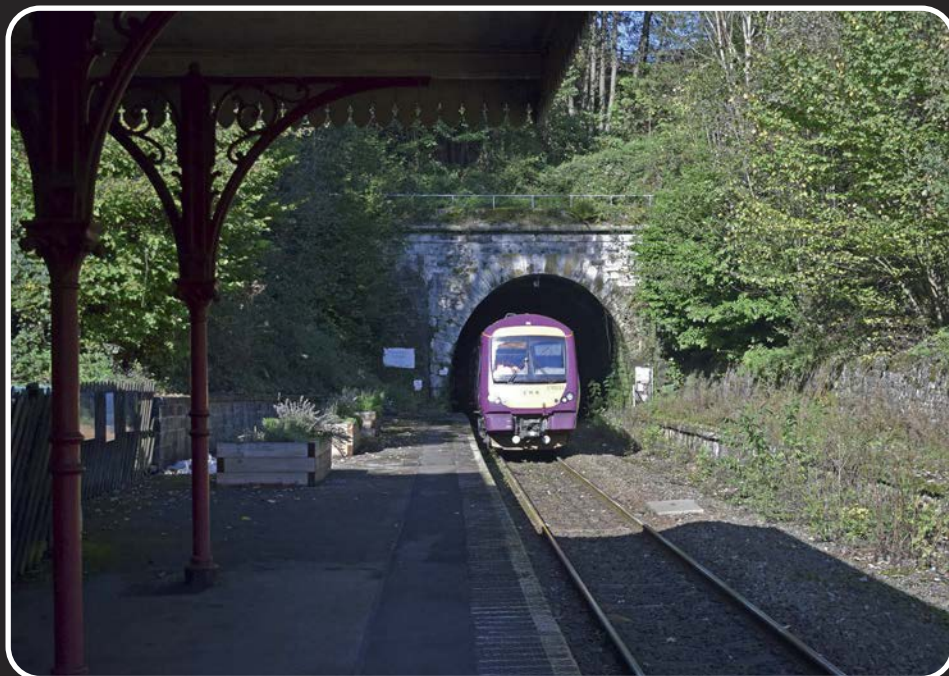
The platforms of Cromford Station, on the truncated line from Ambergate to Matlock Town, adjoin the eastern portal of Willersley Tunnel. It was once a double track bore prior to closure of the main MR Derby-Manchester line.
