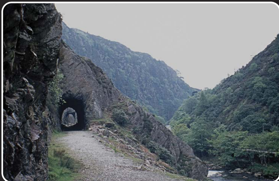
Where trains once passed. Who would have believed in 1976 when walking through this unlined tunnel in the Aberglaslyn Pass that Welsh Highland trains would return?
