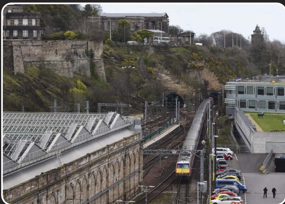
Looking towards the easterly approach to Edinburgh Waverley Station, are the semi-circular portals of the two Calton Hill Tunnels. The earlier bore of 1846 is to the right of the picture and that of the slightly longer, latter tunnel to the left.
