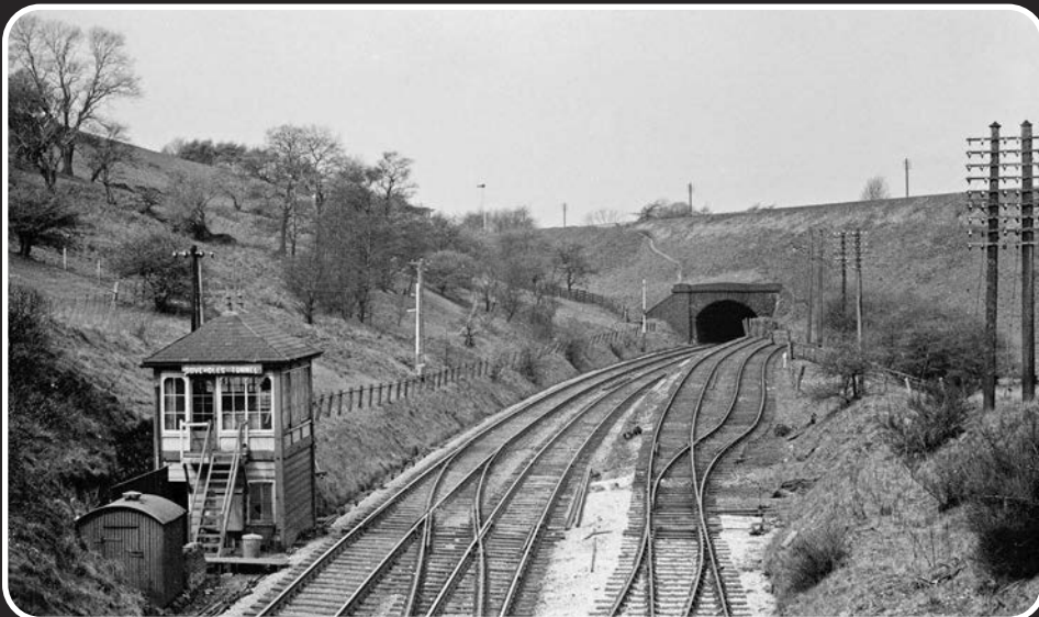
Although the sign on the Midland-style signal box reads 'Dove Holes Tunnel' the portal in this image belongs to the 'LNWR' Tunnel; driven beneath the ex-LNWR line between Buxton and Manchester. The short 95m long bore has segmental arches. The LNWR line passes above the tunnel. Note the signal to the left, while mostly obscured by trees behind, a small part of Chapel-en-le-Frith signal box.
