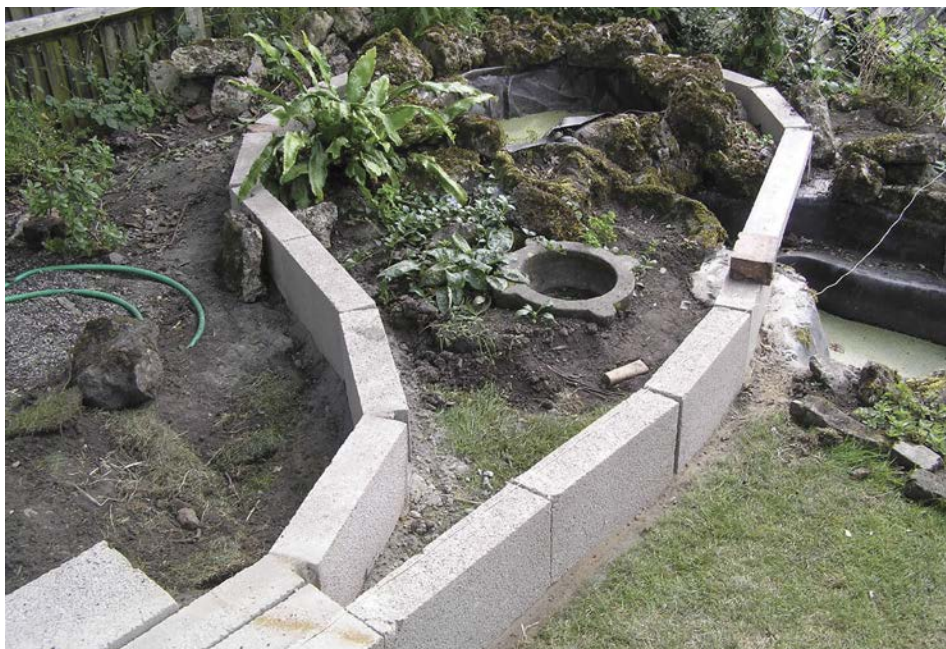
The blocks were reinforced with rocks and the gaps filled with soil to provide planting opportunities. Planting started almost as soon as the slabs were laid, no time to waste.
