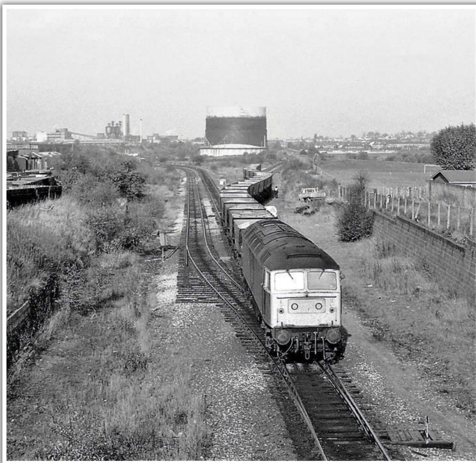
October 1982: An unknown Class 47 performing the empty MGR reversal manoeuvre at Cannock Road Junction shows to good effect the rationalised track layout, which dates from January 1970 (there were once extensive sidings in this area for the stabling of empty coaching stock). This was once the approach to Wolverhampton Low Level station for trains from the Shrewsbury and Stafford directions. The line continuing straight ahead and curving round to the left was once part of the GWR main line from London Paddington to Birkenhead Woodside. SIMON DEWEY
