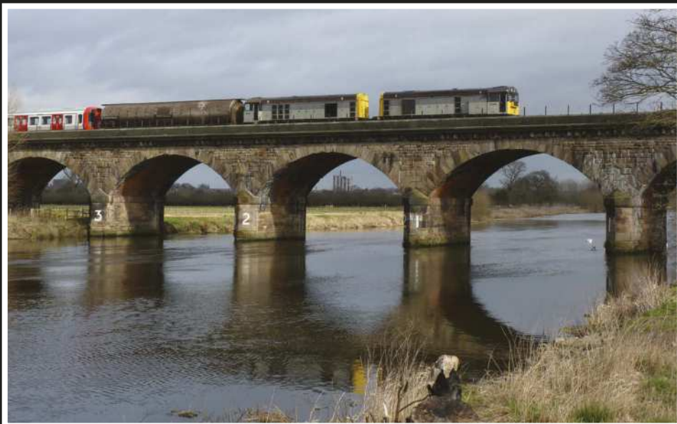
Drakelow Viaduct carries the ex-MR line from Burton upon Trent to Leicester across the River Trent; opened in 1849, the five 'segmental' arches featured in this image are just one of three portions that make-up an approximate ¾ mile stretch that crosses the wide, shallow flood plain. To the extreme left of this image is one of four pill boxes added to the viaduct as a defence against invasion in 1940. Short in height, this stone-built viaduct bears the hallmarks of MR construction. The geometry of a segmental arch is often favoured when designing a shallower structure as a greater headroom can be achieved within the width of the arch.
