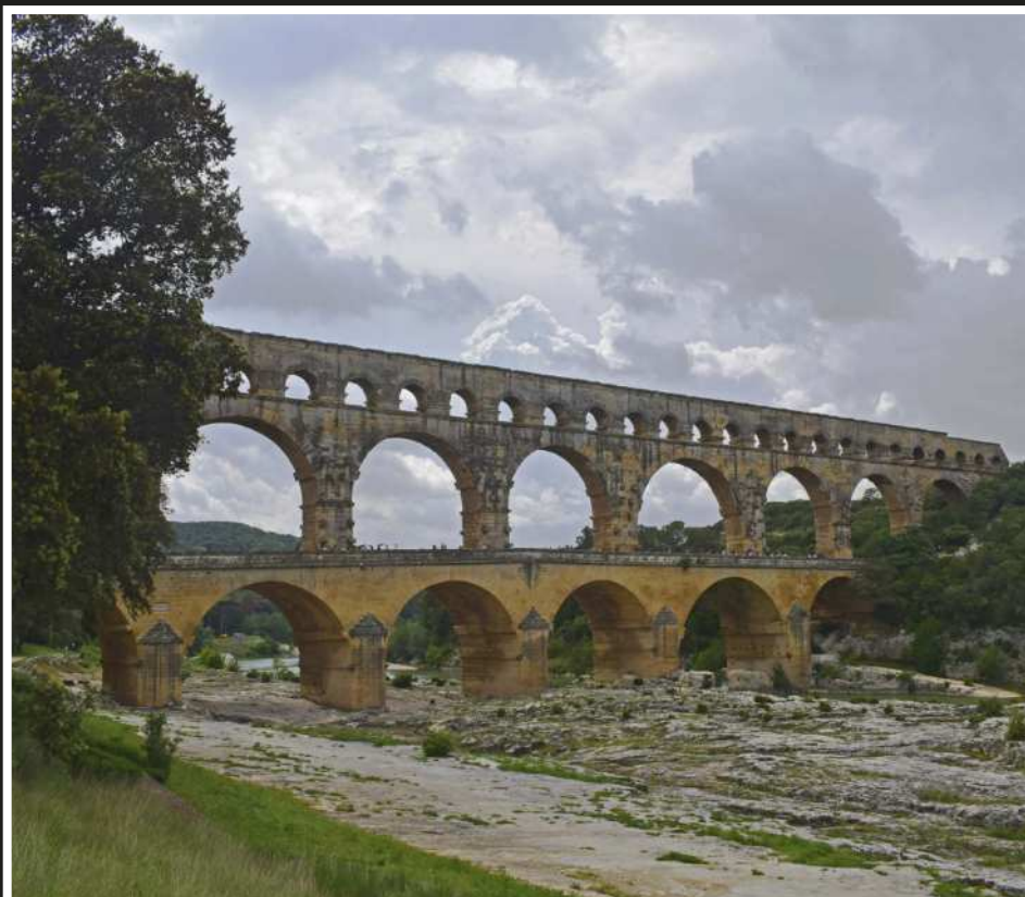
Pont du Gard, originally constructed by the Romans to carry an artificial water course across the Gardon River in France, remains a World Heritage Site. Its three tiers of arches, 273m in length, rise to a height of 48m.
