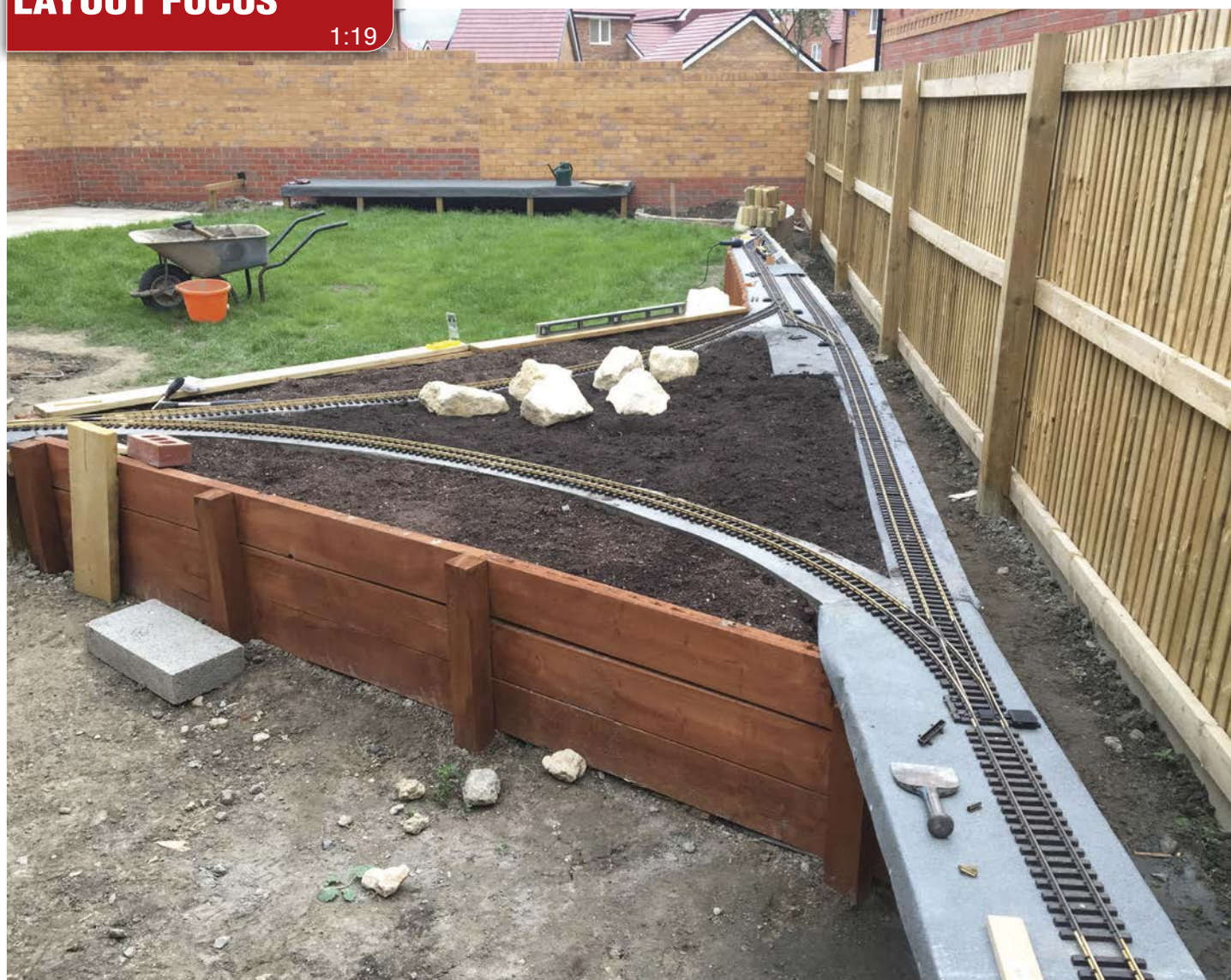
The triangle structure complete and track being laid in July 2017, showing how the walls for the track fit within the wooden structure, prior to planting.
