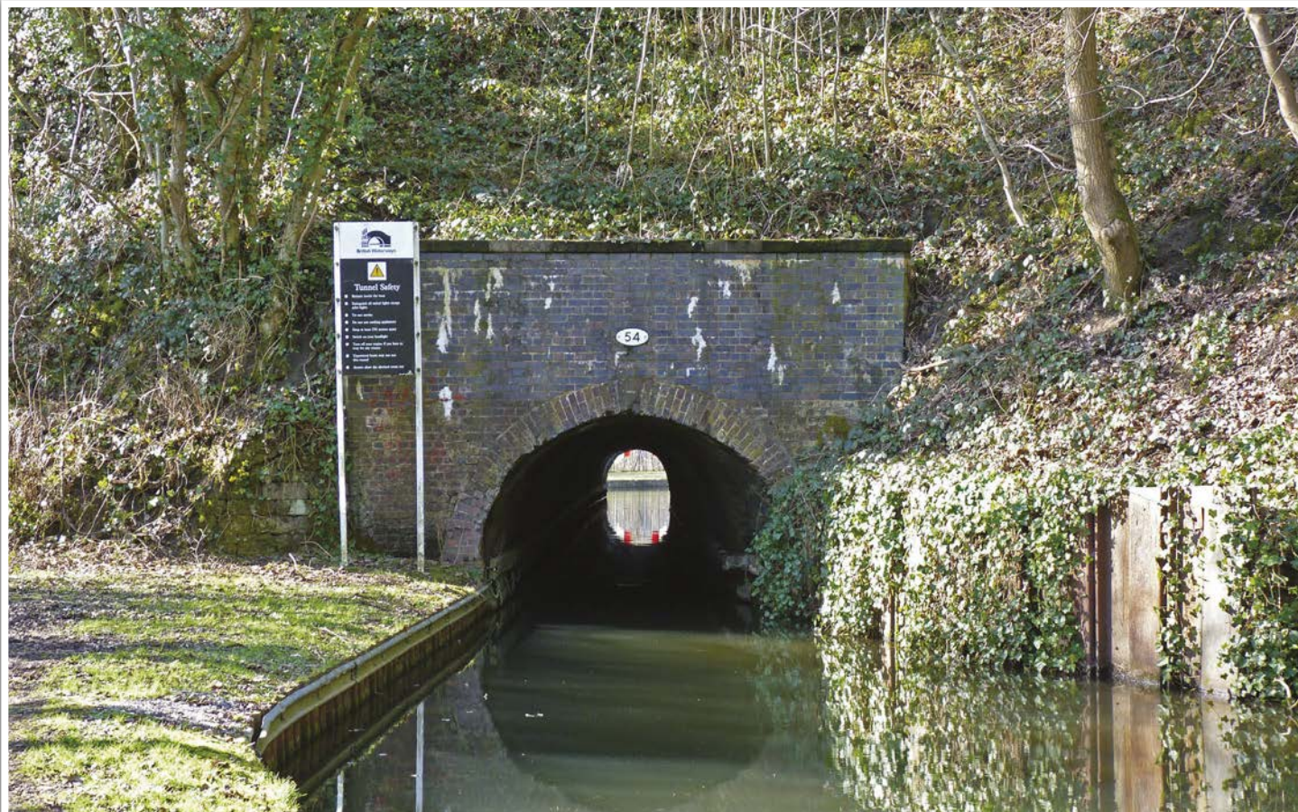
A short tunnel giving access to Frogall Basin. Frequently found on hilly routes, the tunnel didn't accommodate a tow-path, and the boaters would have to 'leg it'. Laid on their backs on the cabin roof, their feet would push along the tunnel arch.
