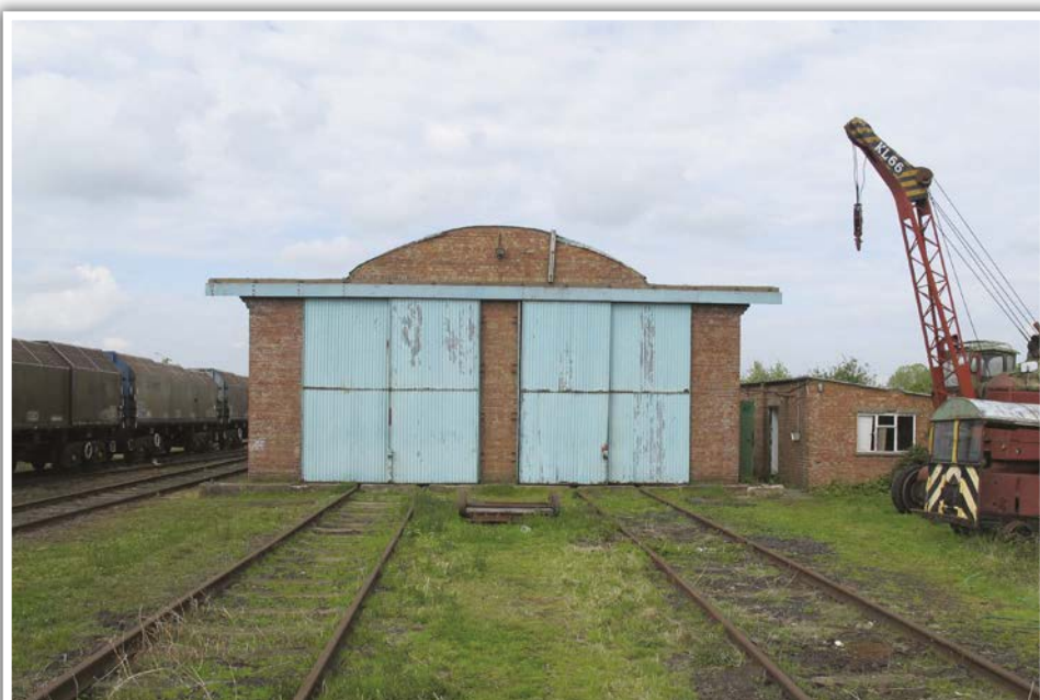
Engine maintenance shed on Long Marston depot's railway – a hybrid between a Nissen hut and a shed that whets the modeller's appetite. Source: PHIL PARKER
