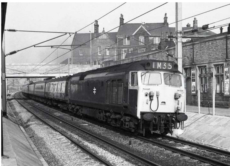
Part of modernisation involved taking Carnforth's WCML platforms out of use to permit track realignment for higher speed. On 30th March 1974 50009 sweeps through the former platforms with 1M35, the 13:55 Glasgow-Euston that was booked for a pair of '50s'. DAVID CLOUGH
