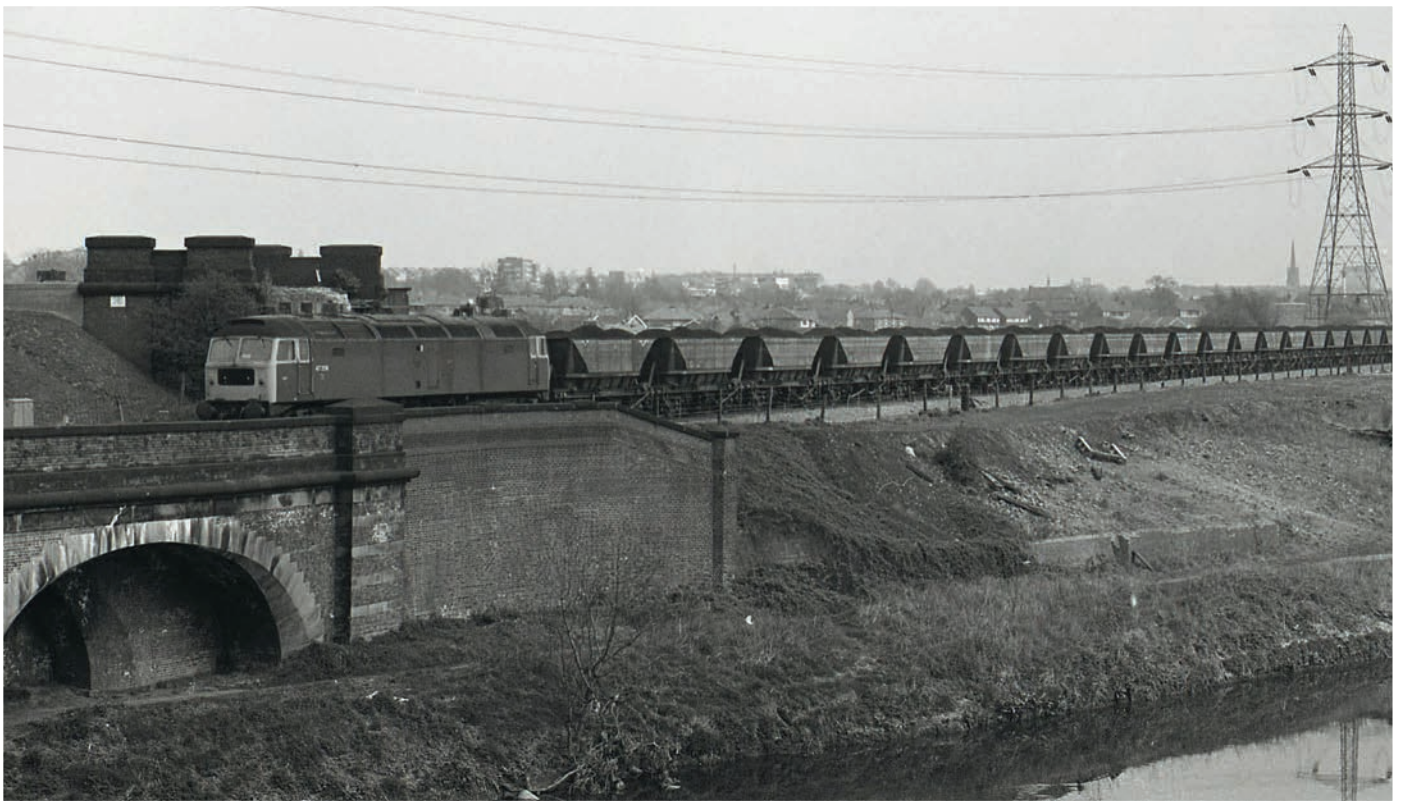
This view at Heaton Mersey in north Stockport includes the River Mersey and the abutments of the former Midland Railway viaduct that carried the Manchester Central to New Mills South Junction route across the valley. 47228 and its load of coal for Fiddlers Ferry Power Station from South Yorkshire approach Cheadle Junction on 24th April 1980. Heaton Mersey shed was on land out of shot to the rear of the train. DAVID CLOUGH
