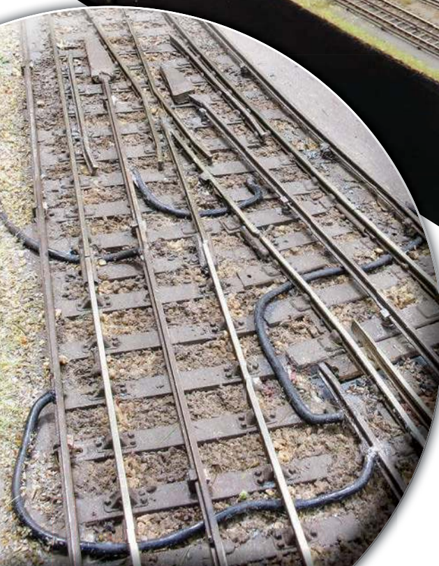
Typical three-rail LT trackwork at the entrance to the depot.
