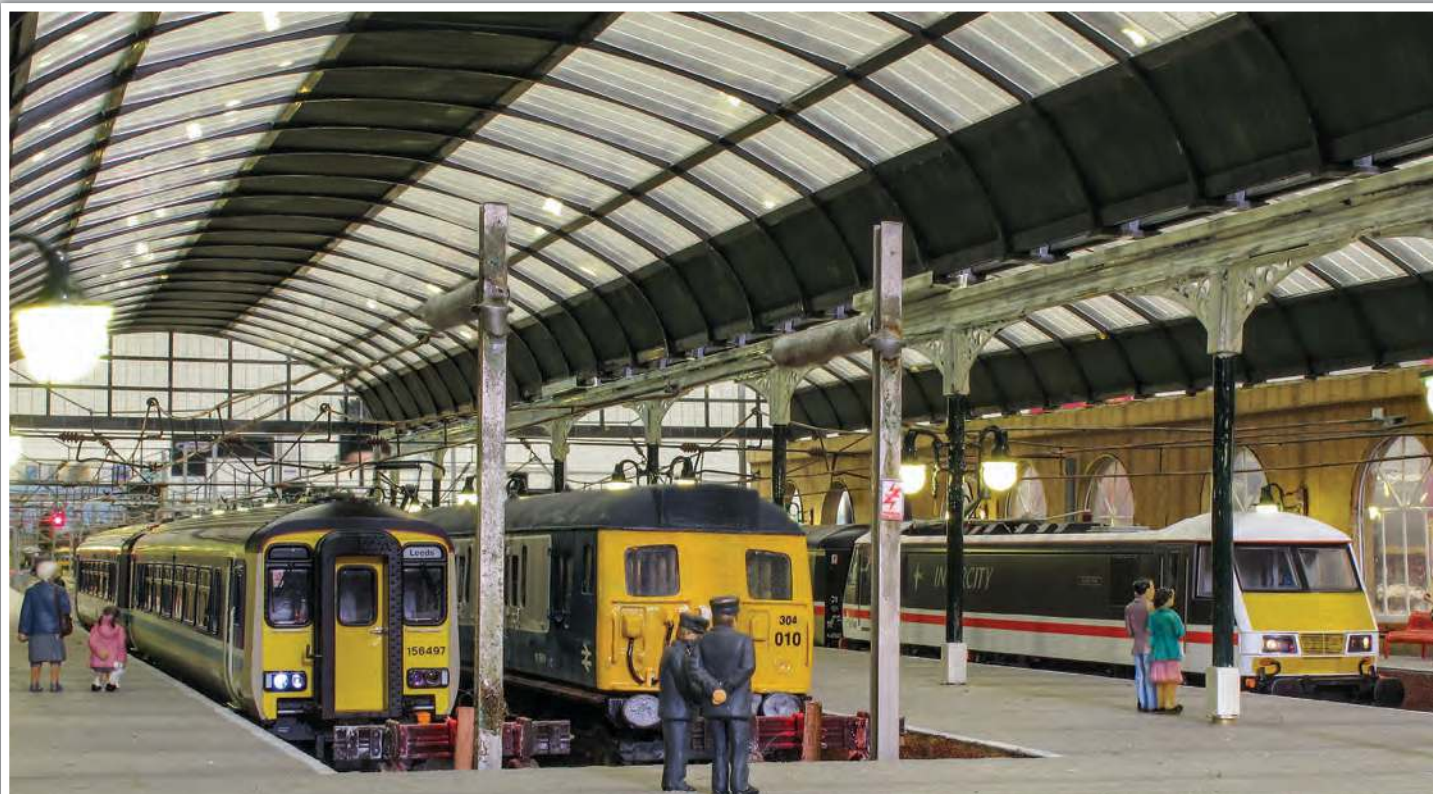
A view not normally seen by members of the public at exhibitions; this is the sight that you would be greeted with having just walked through the station entrance on to the platforms. A Class 156 DMU service for Leeds occupies platform 4, a Class 304 EMU on a service to Crew on platform 3 and Class 90 90005 on platform 2 with the arrival from Birmingham.
