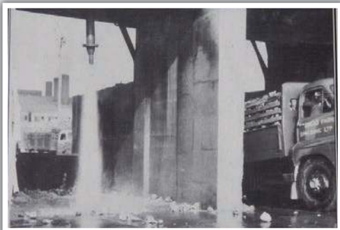
The high-pressure hose operated from a cabin above washed the beet from lorries that weren't able to tip. The beet was washed along a flume to a storage area.
