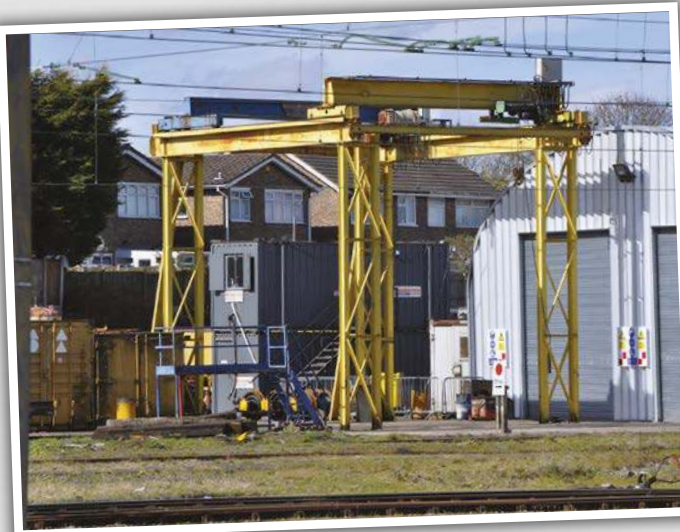
Overhead gantry crane and blue inspection platform at Bescot. Note the shed to the right on which the layout drew inspiration.
