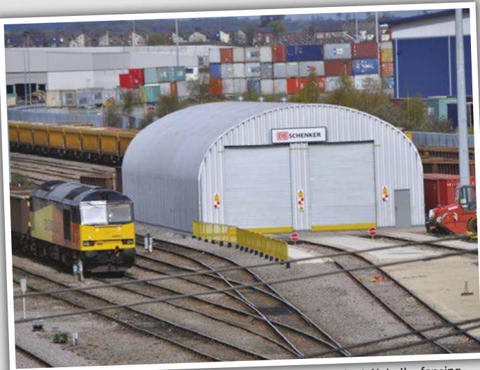
The distinctive parabolic roof of Doncaster wagon repair shed. Note the fencing.
