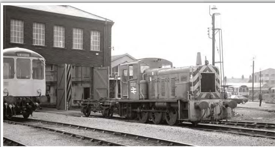
ABOVE: In 1958 Hammerton Street diesel depot, which was located just outside Bradford Exchange station, was converted from the old Great Northern Railway steam shed to maintain DMUs and diesel shunters. In this view, 03371 is stabled outside the depot on the August 11, 1978 in the company of a Class 104 and a 'Calder Valley' Class 110 DMU. The depot closed in 1984. DAVE HIGSON
