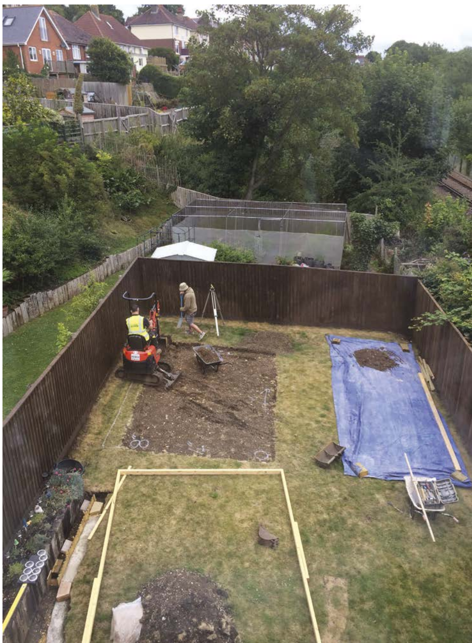
Ensuring level foundations.
