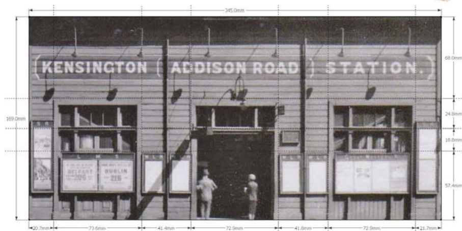
Dimensioned photograph of the down station booking hall.
