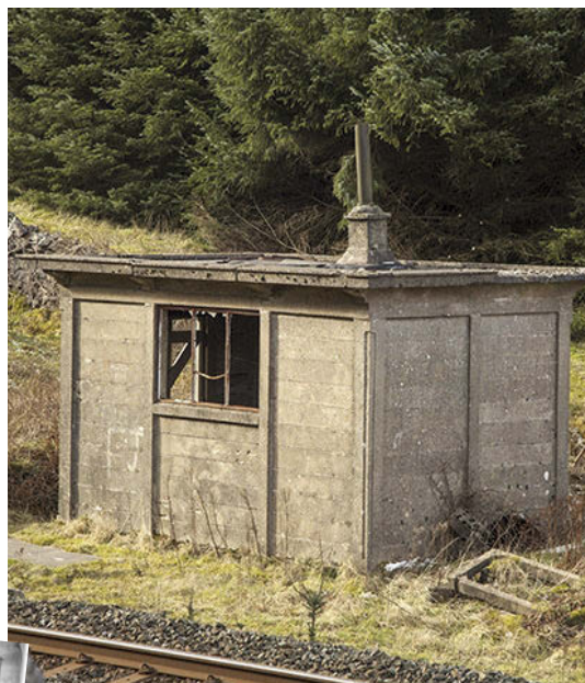
Three views of an LNER-style modular concrete hut near Garsdale on the Settle to Carlisle line. Note the uprights, into which the concrete panels are slotted - even the chimney base is made of cast concrete. The minimalist design with a felt roof is an ideal candidate for modelling.
