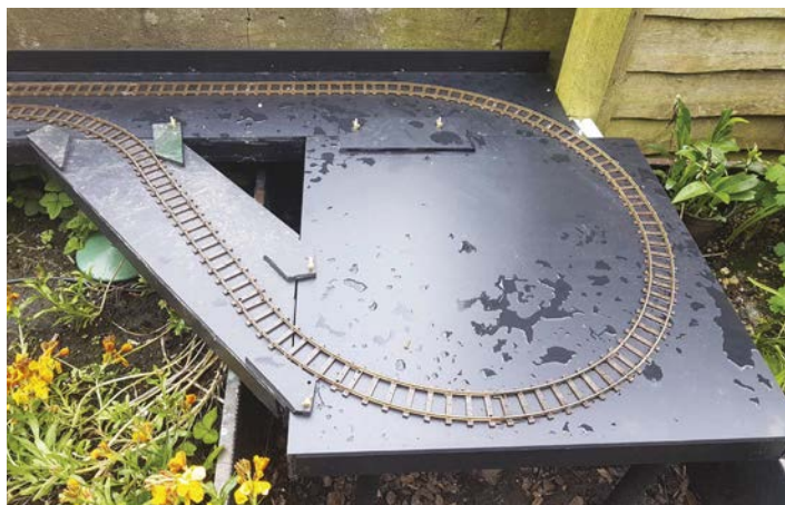
Above: The loop and diagonal boards tapped for support and bolted in.
