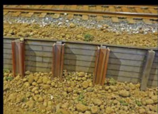
MW10003 Timber retaining wall
