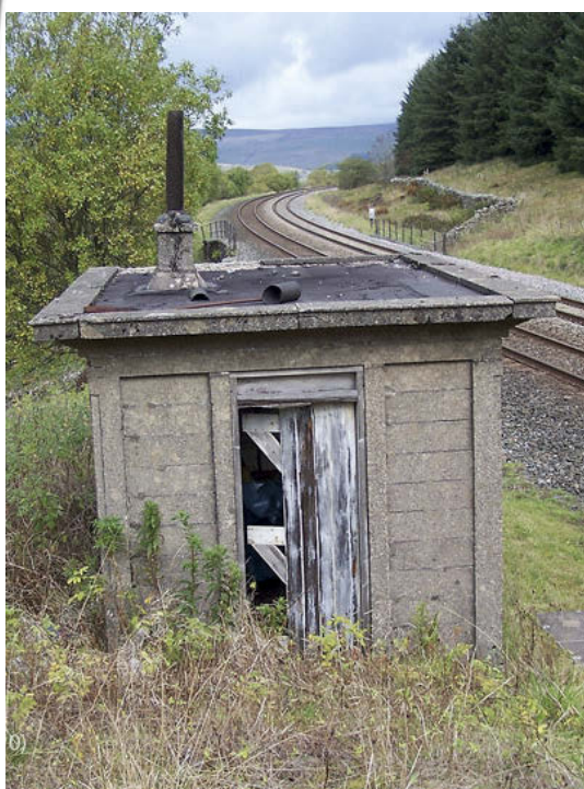
Three views of an LNER-style modular concrete hut near Garsdale on the Settle to Carlisle line. Note the uprights, into which the concrete panels are slotted - even the chimney base is made of cast concrete. The minimalist design with a felt roof is an ideal candidate for modelling.
