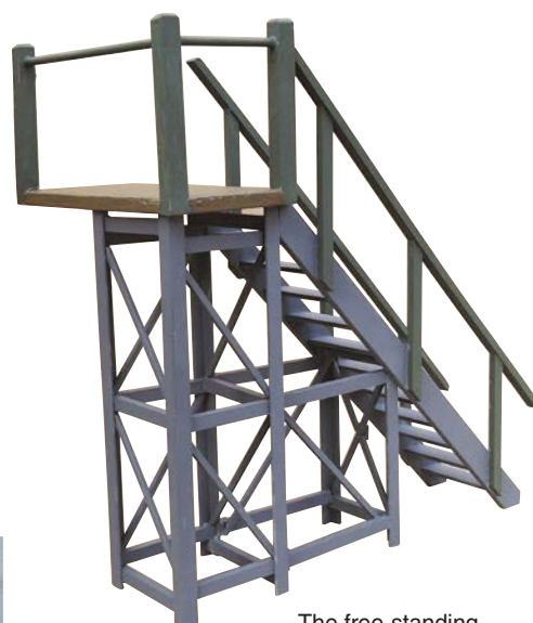
The free-standing section of the fire-escape.
