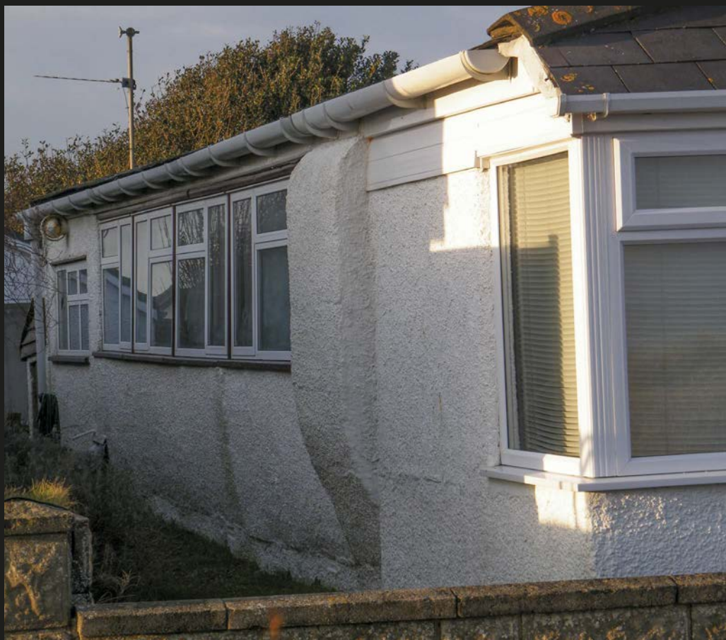
A side view of a carriage at Pagham in West Sussex. They're easy to spot from the beach, normally in pairs and the gap between is filled with extra living space. The carriage doors and windows down the sides of this example have been cutout and replaced with uPVC windows. Conveniently, the guard's observation post has been 'dashed over' – possibly a post Victorian LSWR coach? You could model this example and place it on a present-day era layout. CLIVE BARKER
