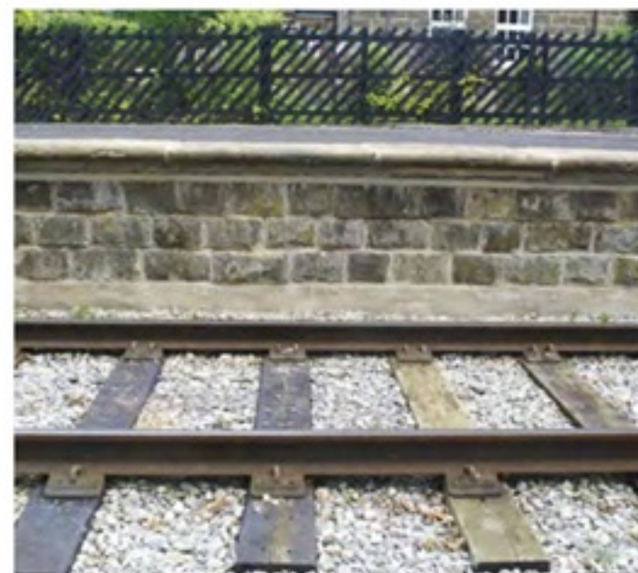
This photograph, taken at track level gives a good view of the station platform walling, edging stones and the diagonal Midland Railway design of fencing at the rear.
