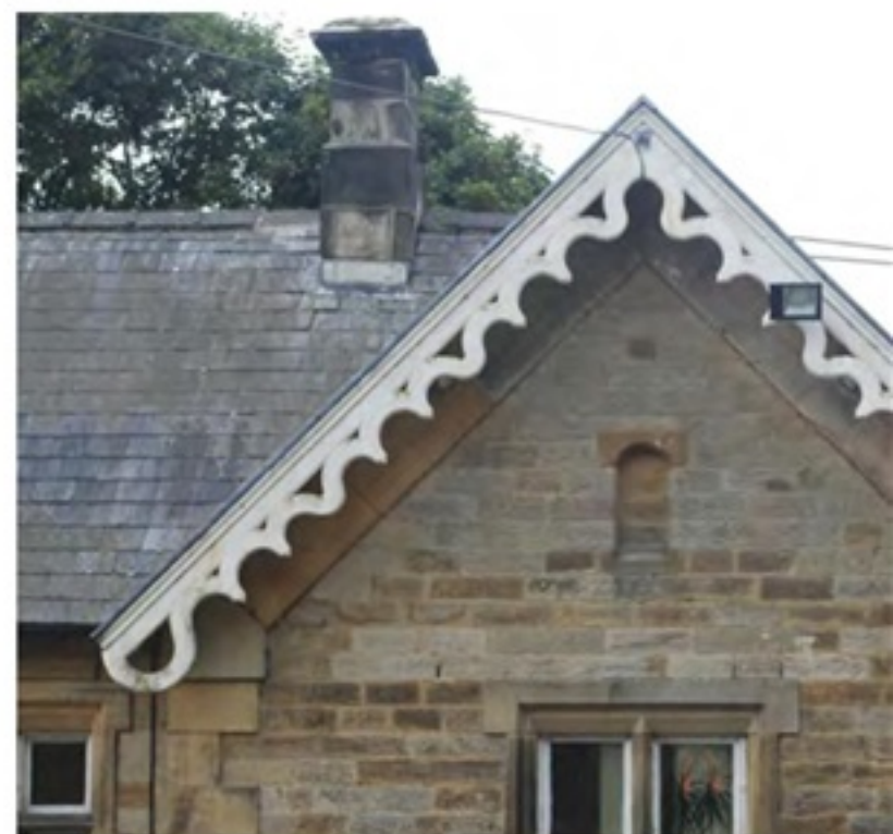
I have included the yard view of one of the gables to show the design of the barge boards. With the camera angle at a higher position, the barge boards could be used to scan for laser cutting ready to use on a model. The rain staining to the roofing slates is also clearly evident in this image.
