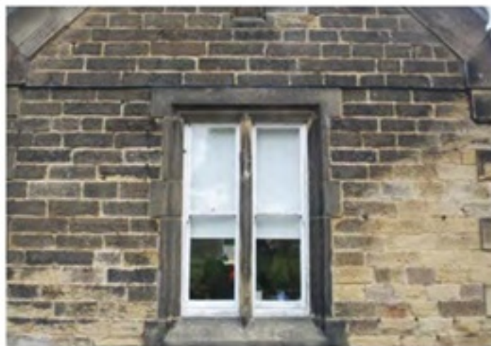
I have included this image to show the main window detail, consisting of stone mullions. It also gives good colour reference to the weathering of the stonework.
