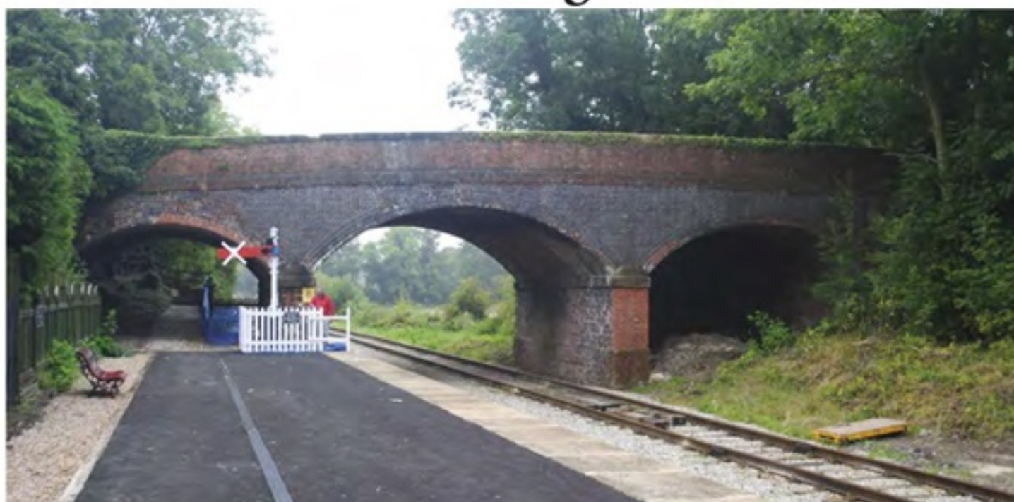
This photograph shows the over bridge carrying the A517, Belper to Ashbourne trunk road. The over bridge at Hazlewood is almost identical to this one at Shottle, using blue and red brick for construction.
