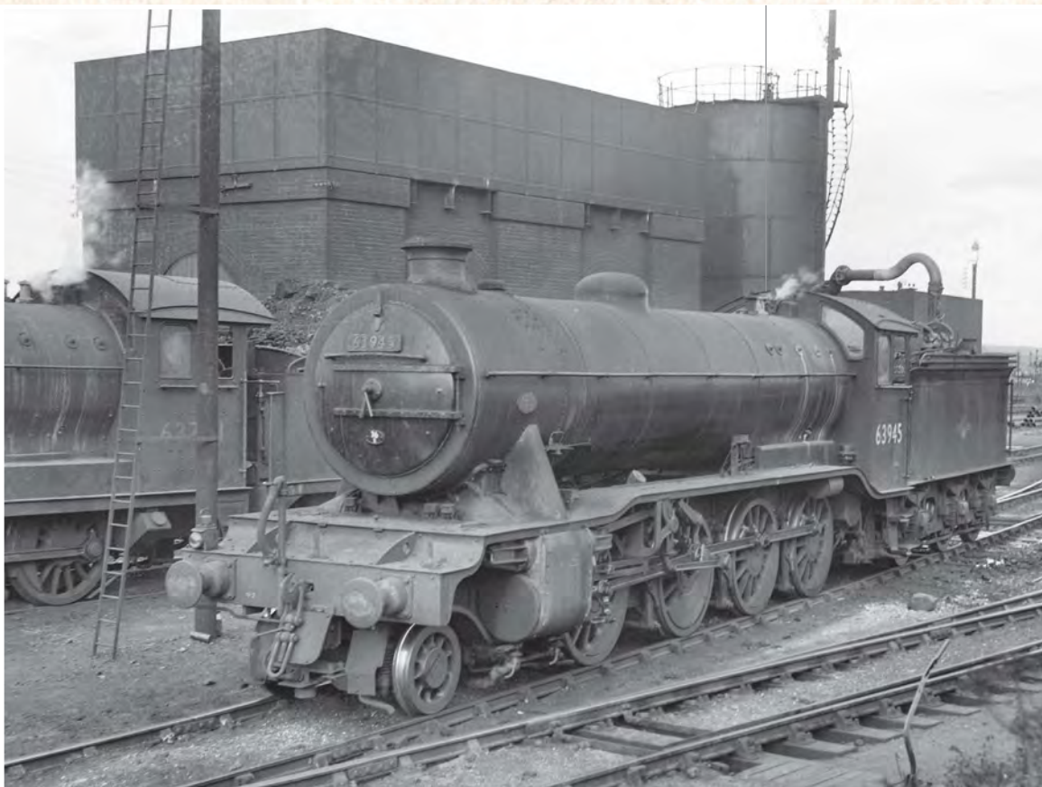
Another variation on the O2/4 theme takes water at Frodingham shed in Scunthorpe on September 26 1959. No. 63945 has been rebuilt with an LNER 100A boiler (like the O4/8 alongside) but retains a GNR style tender.
