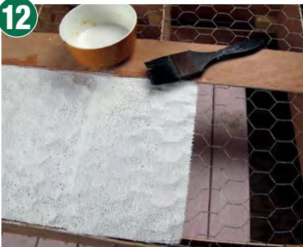
Cut the material to length whilst it's dry, then dampen with water using a paintbrush. Overlap each piece by an inch.
