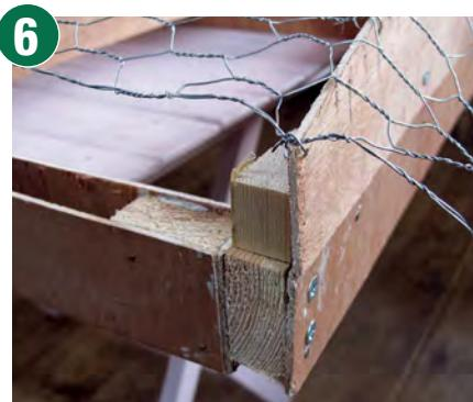
Spread your chicken wire over the baseboard and drill holes around the edges and across the formers that marry up with the mesh size employed.
