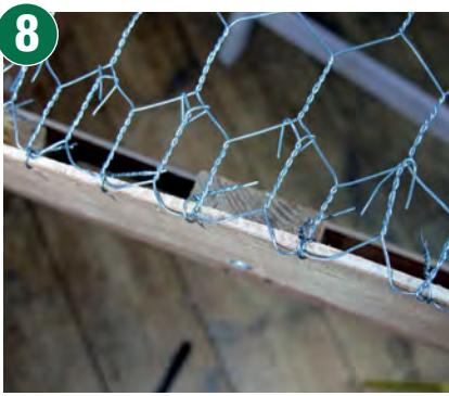
When the mesh is secured, cut off any overhang and fold the end back to strengthen the outer edges.
