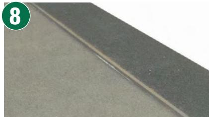
The sides of the plastic strip that face the road surface and the edge of the pavement have a trace of latex adhesive applied and are then carefully positioned. Don't worry if there is excess glue as it can be wiped away. Any residue will be transparent.
