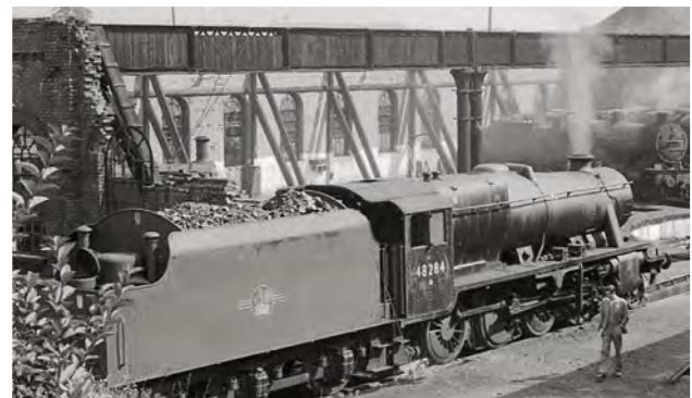
There's substantial structural variety. Of note is the partial gable end with exposed window frame nearest the camera, contrasting the full gable opposite. A series of wooden buttresses make a clear statement about the condition of the left hand wall. Visiting locomotive, Stanier 8F No. 48248 takes centre stage in this 1960s view.
