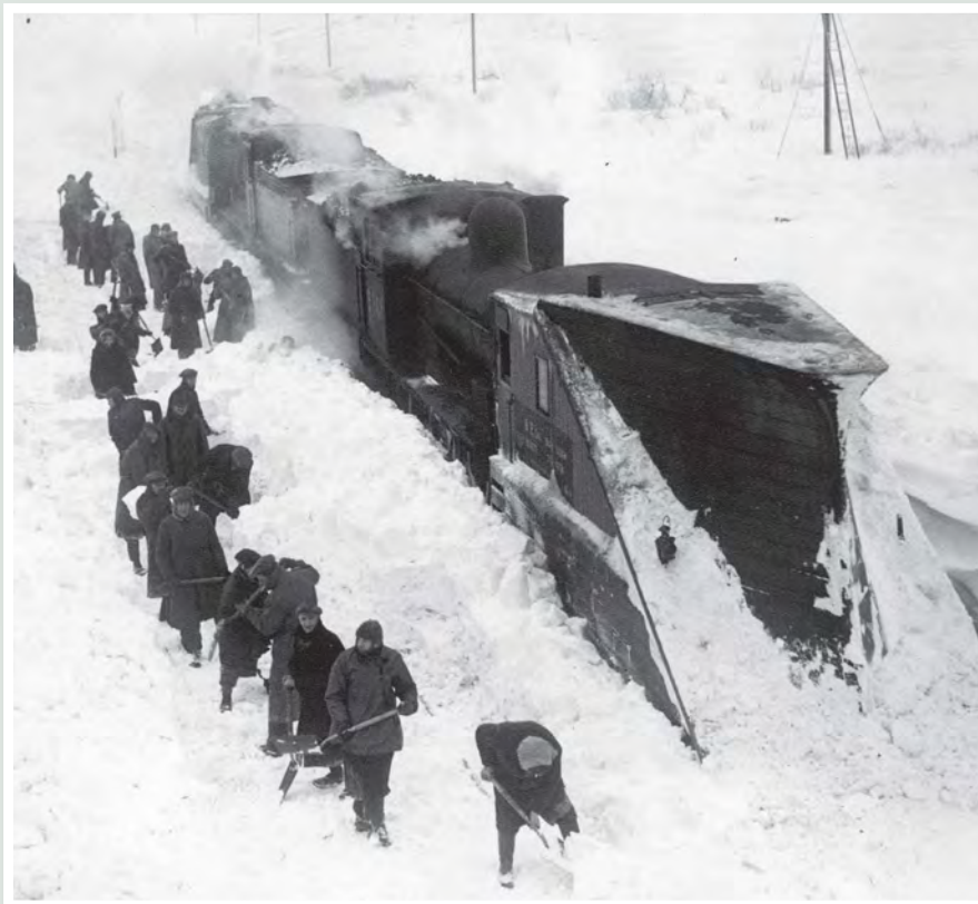
In the famous winter of 1947, PW men clear the line manually at Stainmore Summit, 1,370' above sea level (the metal summit sign is just visible top right). A pair of J21 0-6-0s simmer between the two former North Eastern Railway snowploughs that are carving a path through the deep drifts. KEN HOOLE STUDY CENTRE
