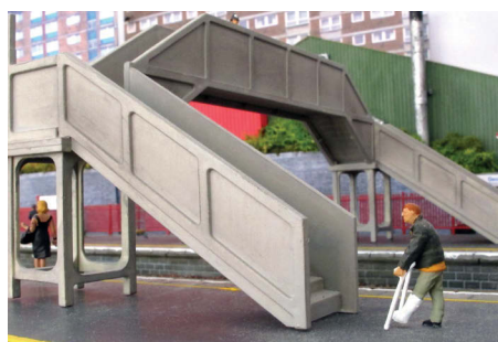
The footbridge looks particularly imposing today!
