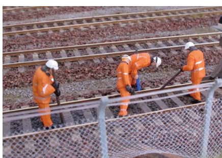
Track workers working fast to repair a siding.
