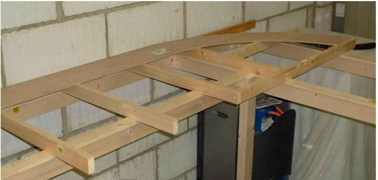
An L-girder construction layout being installed in a garage. The fixed supporting leg can be seen in the corner of the front. The rear 'L' members are turned to face into the centre of the layout and securely fixed to the wall. A flat track bed of 9mm ply has been partly laid onto the joists and is waiting for the connecting sections to be added before track laying commences.
