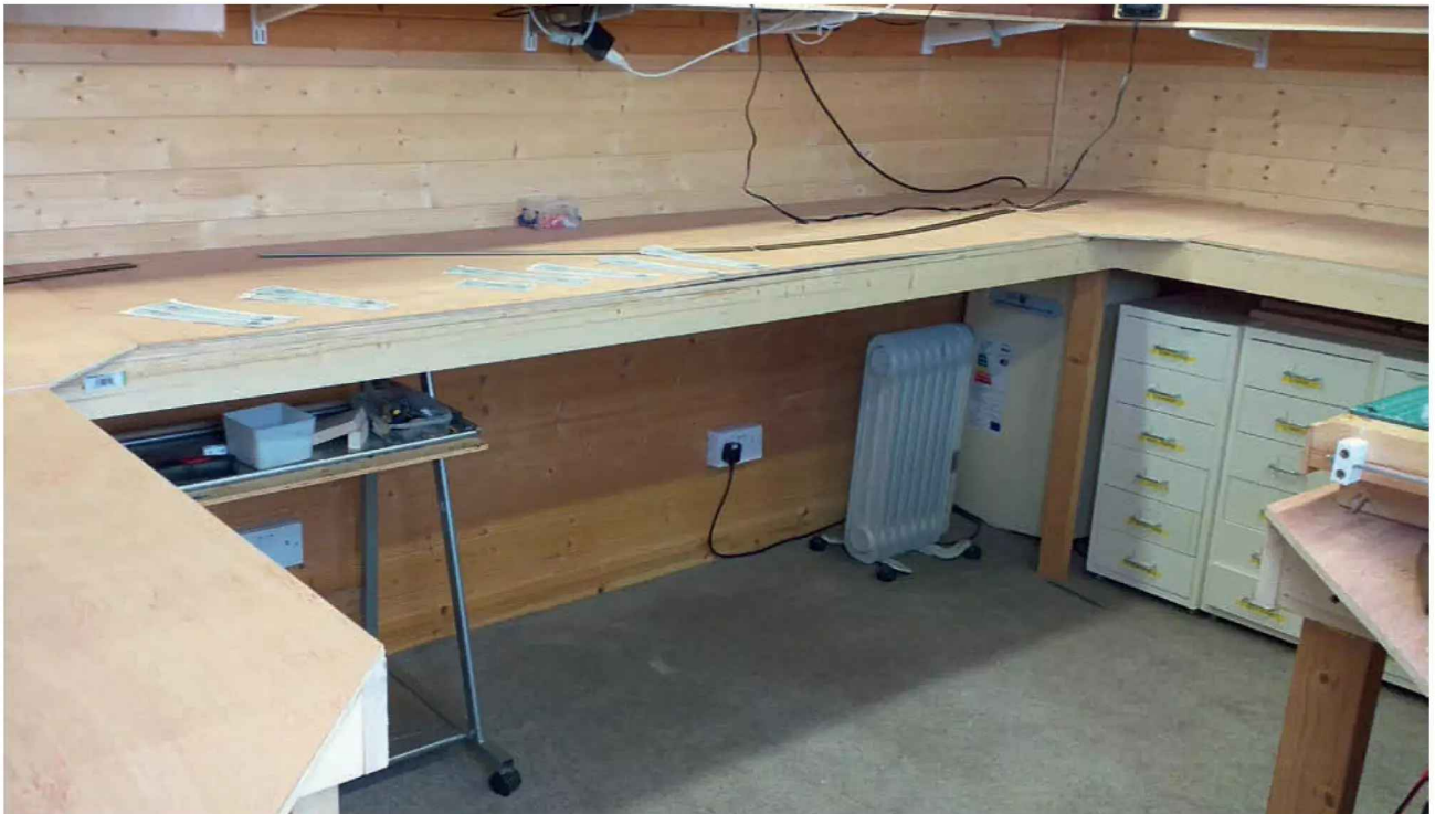
Another garden shed that has been insulated and had all the walls, ceiling and floor lined, plus good overhead lighting and mains power sockets have been installed. Image courtesy of Steve Mumford
