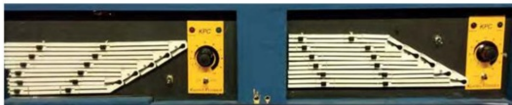
Above Fleischmann switches were used to create a mimic board for operating the points and isolating sections.
