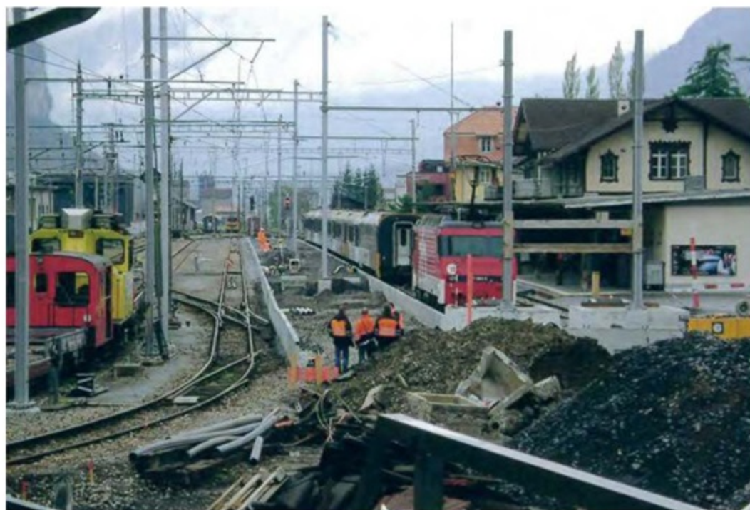
Below April 2010 – rebuilding the Zentralbahn station, showing the shell of the new island platform. Note the curving connection to the MIB.
