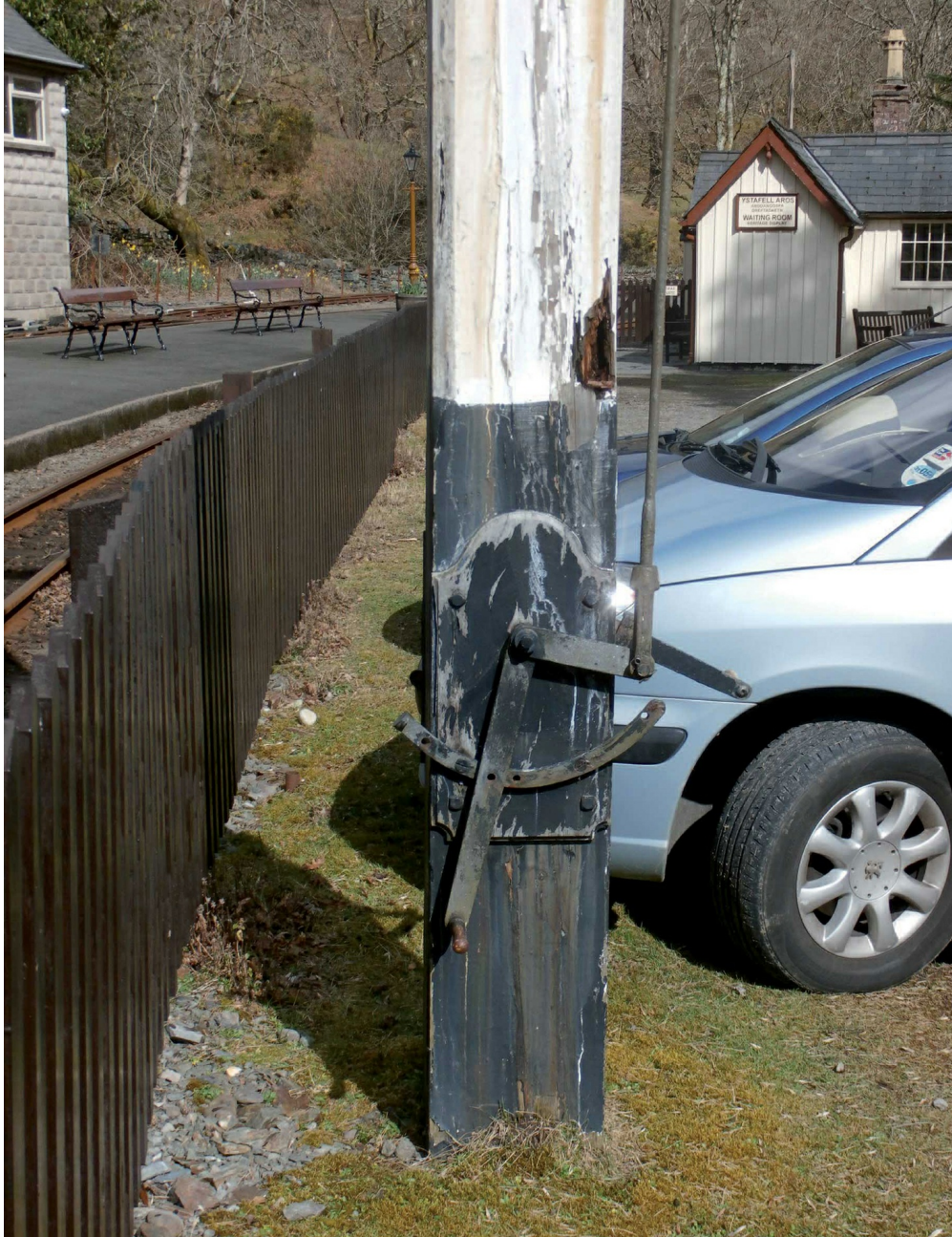
Detail of operating handles for the split-post signal.
