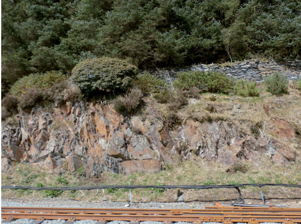
Rock faces contain large amounts of red/orange/oxide colour (compared to the slate wall above in this shot) and the strata are almost vertical.
