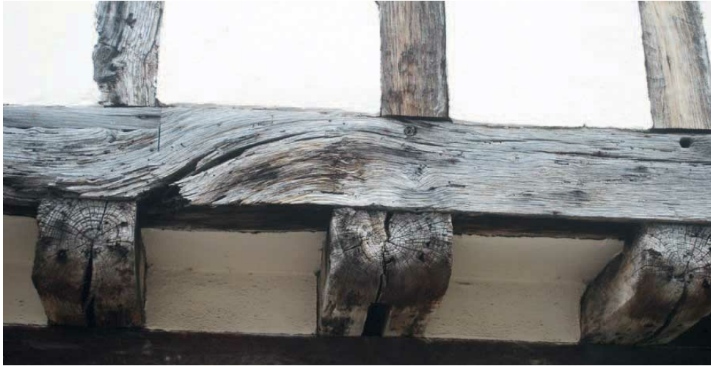
The timber frame and the timbers forming the jetting beams to support the wider upper floor.
