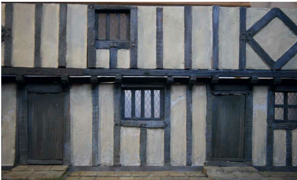
The lower side of the building now connected with the upper side. Note how the upper side is sitting on the jetting beams, also the decorative diamond
