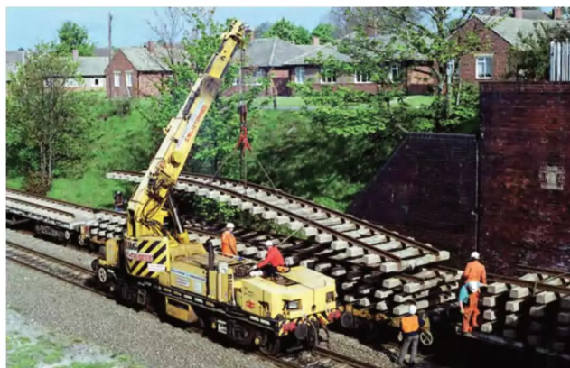
ABOVE: The most recognisable of all the Civil Engineers cranes is the telescopic jib Plasser & Theurer GPC-72 design, DRP81503-32 being delivered between 1977 and 1981. With some still seeing use with Balfour Beatty, they could handle most jobs, including lifting track panels as DRP81527 displays at Horbury in May 1991. The sagging of the 60ft track section also illustrates why track relayers were preferred for such jobs. David Ratcliffe
