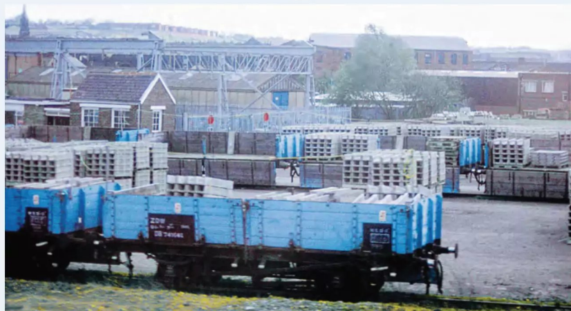
LEFT: Although of indifferent quality, this image of Leeds Whitehall Road taken from a passing train in April 1993 shows Project Mercury in full swing and provides plenty of modelling interest. Numerous 12-ton pipe wagons are present and in the process of being filled with concrete troughing, these being loaded 16 to a pallet and secured with plastic strapping. The wagon on the far right also has a palletised load of troughing lids with approximately 40 stacked in an interlaced manner while the ZDW alongside has a stack of eight empty pallets as a partial load. Simon Bendall Collection
