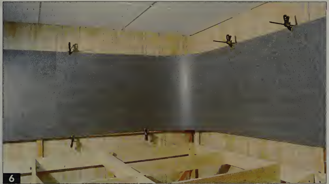
6 Clamp the second sheet of hardboard in place, so it butts tightly against the previous piece, and make sure it is level.
