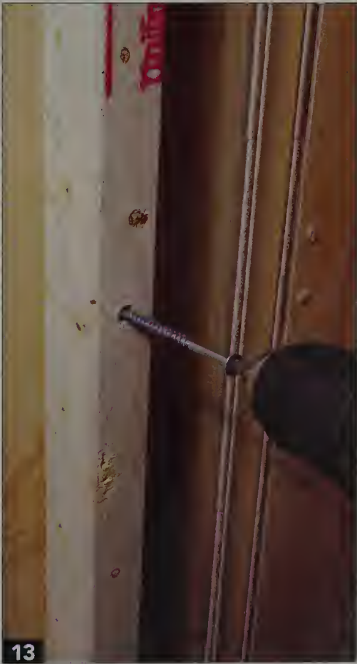
Anchor a vertical 2 x 2 to the wall with screws long enough to securely grab the stud. This is a 3" square-drive deck screw.
