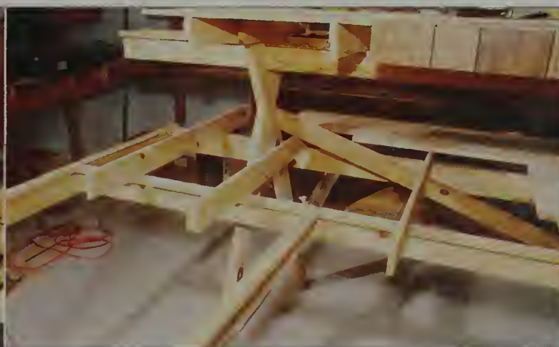
10 Jim Hediger uses a 2 x 4 X-frame design to support L girders on both decks of the freestanding portion of his HO layout. This allows a long span between supports. Jim Hediger, both photos
