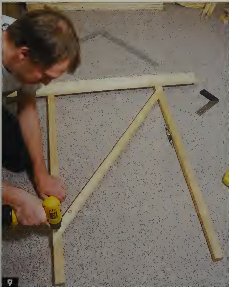
9 Add the first diagonal brace and then flip the assembly over and add the second brace.
