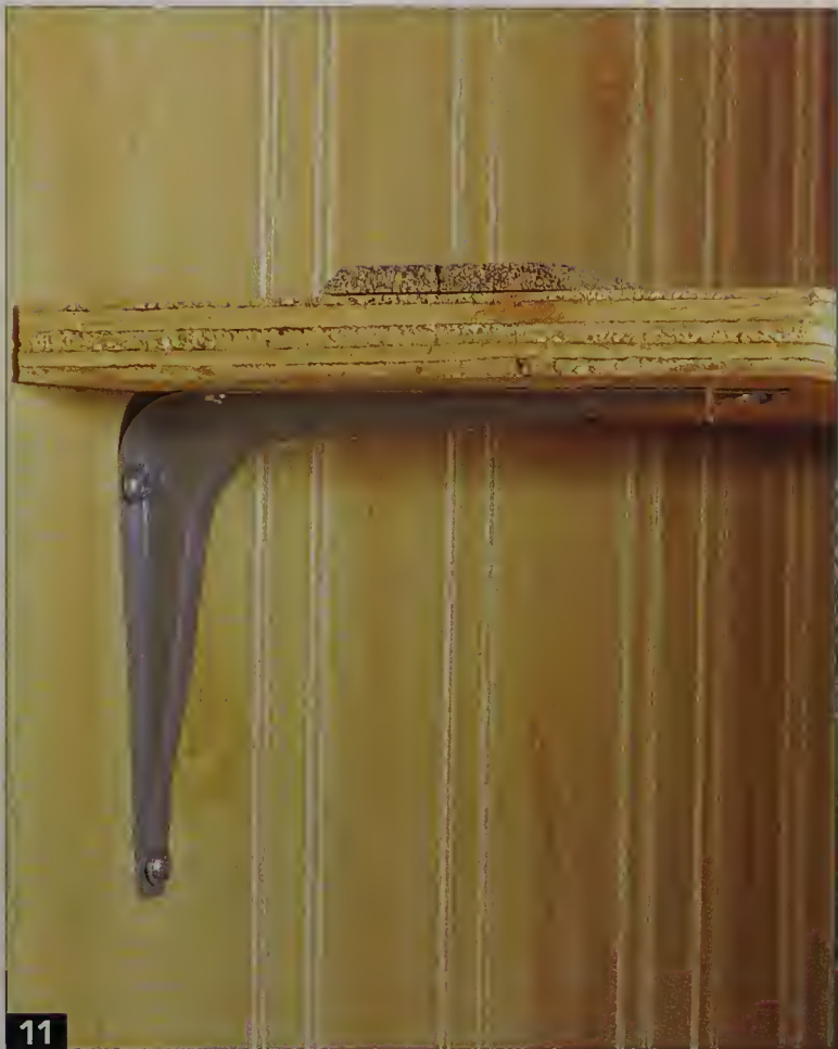
A narrow plywood shelf can be placed directly on commercial shelf brackets as long as it's supported every 18" or less.
