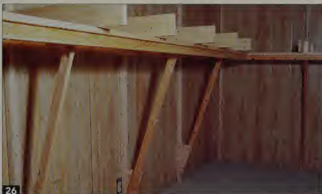
Joists have been added to the girders. The benchwork is ready for roadbed.
