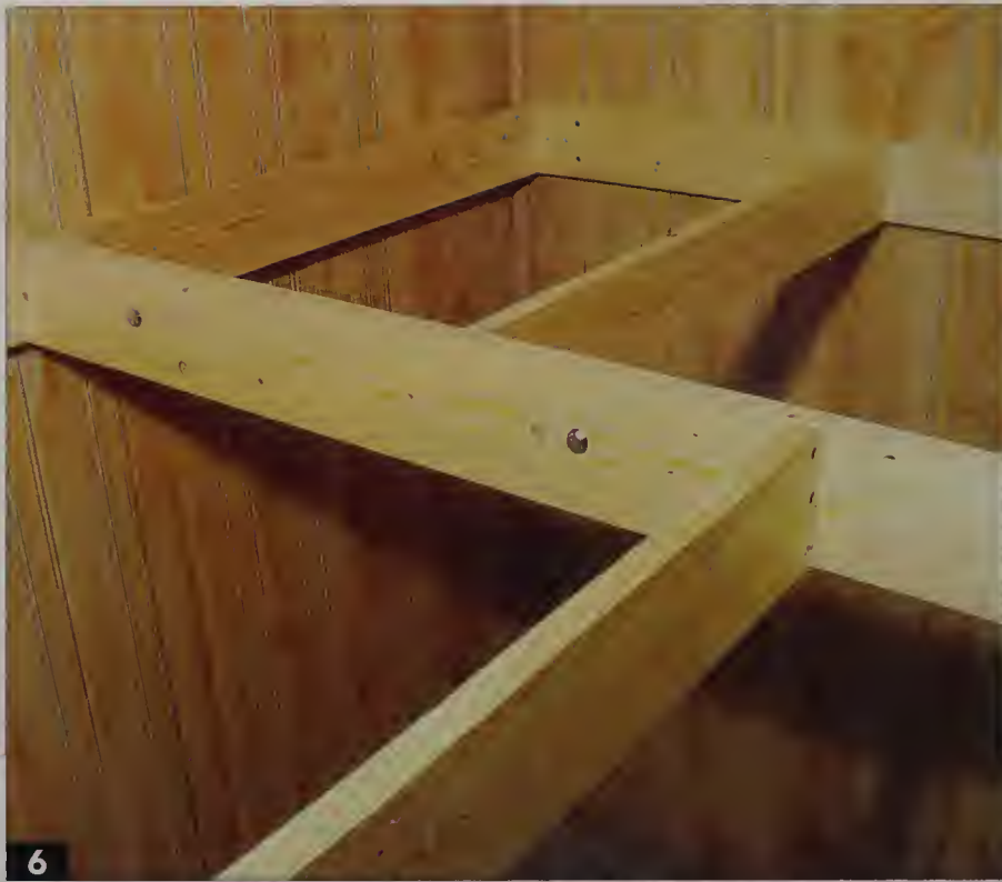
Join the two sections with a couple of carriage or hex bolts.
