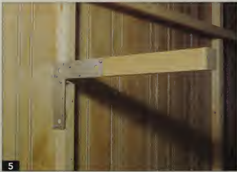
5 Stamped steel L braces work well for supporting 2 x 2 brackets. Use an angle on each side of the bracket.
