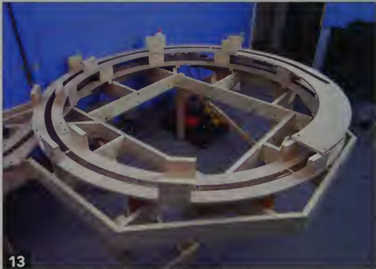
Jeff built a grid table of 1 x 4s with 2 x 2s to support the helix. The roadbed is ½" plywood with 3"-wide spacer blocks between levels. Flextrack is screwed directly to the plywood. Jeff Johnston
