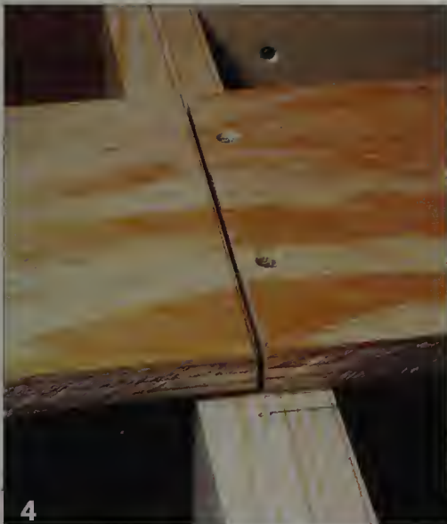
Cut the plywood for the liftout, so there is a narrow gap at each end.
