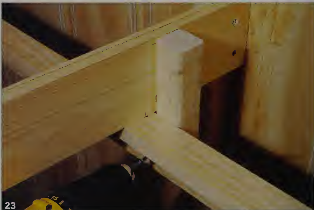
23 Screwing a short 2 x 2 to the girder and bracket will strengthen the joint.
