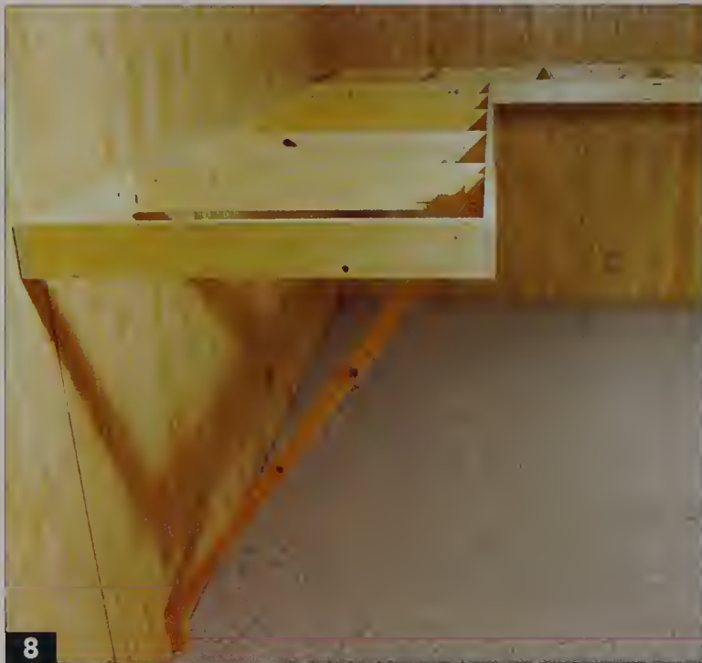
Diagonal braces take up no floor space. A short length of 2 x 2 screwed to a wall stud gives the 1 x 2 brace a solid anchor at the bottom.
