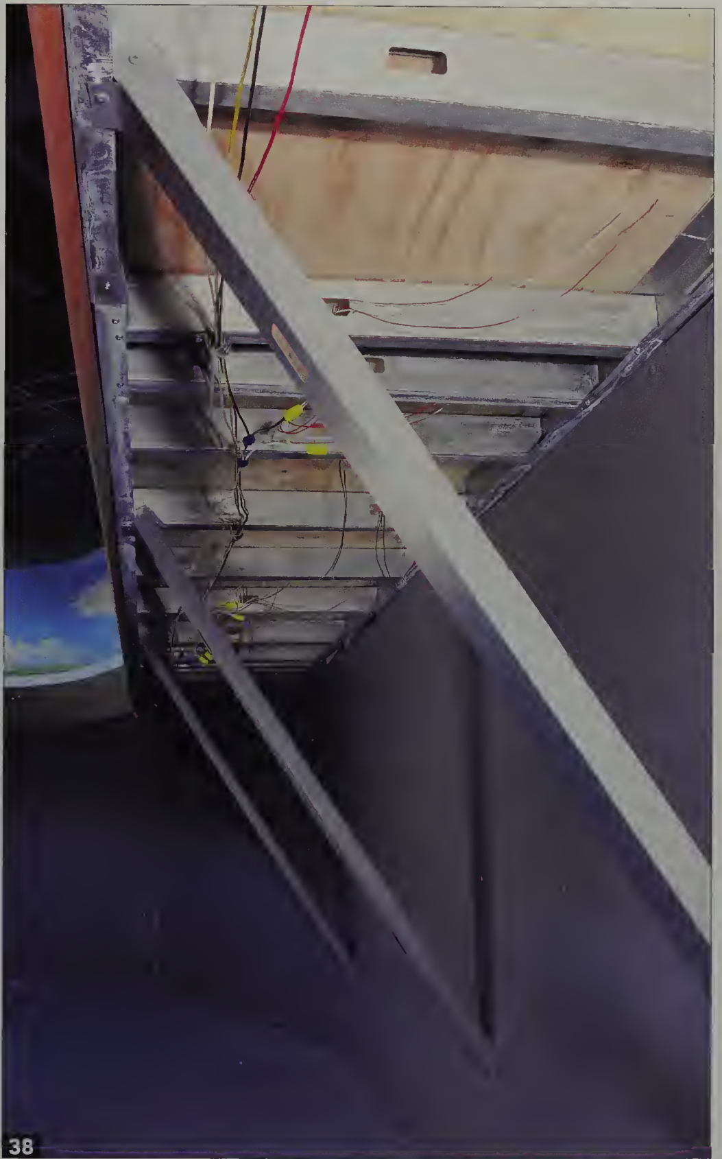
This benchwork grid is made from steel stud cross members screwed to steel tracks. The braces are also steel studs, and the benchwork is topped with 1/4" plywood. David Popp
