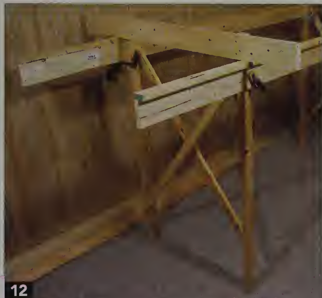
12 Clamp the girders to the completed leg assemblies.
