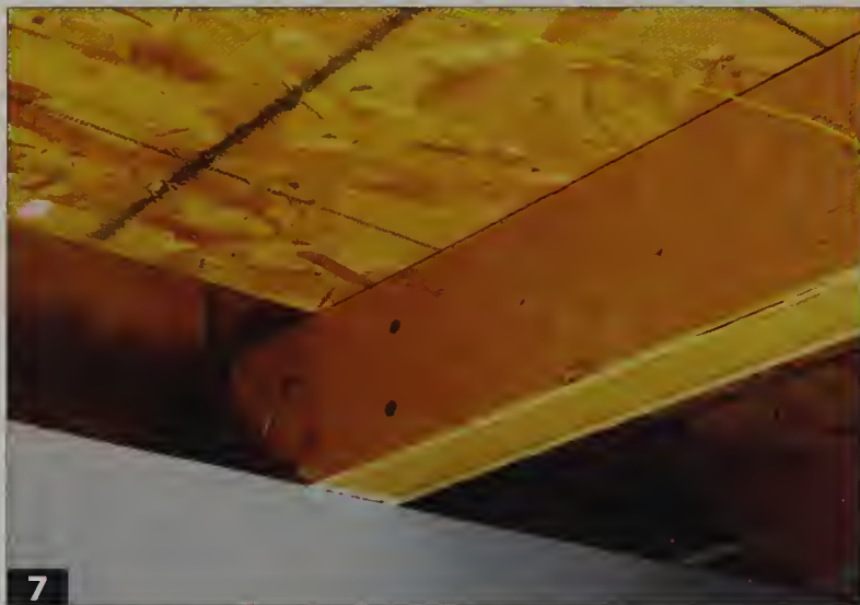
7 Developed by Jim Murphy, this design has the 2 x 4 arm butted firmly to a 2 x 4 wall stud, with a plywood sandwich that is screwed in place. The design is quite stable. Don Meeker
