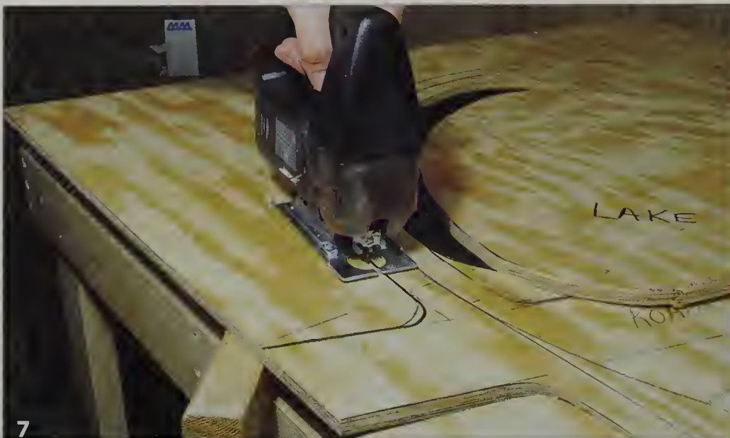
7 Cut the plywood with a saber saw. Use lumber scraps to elevate the table, so the saw doesn't cut the girders.
