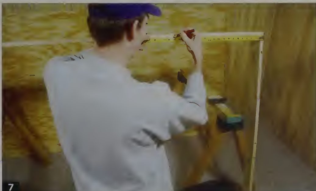
Mark the location of the center of each crosswise joist on the top of each side member.
