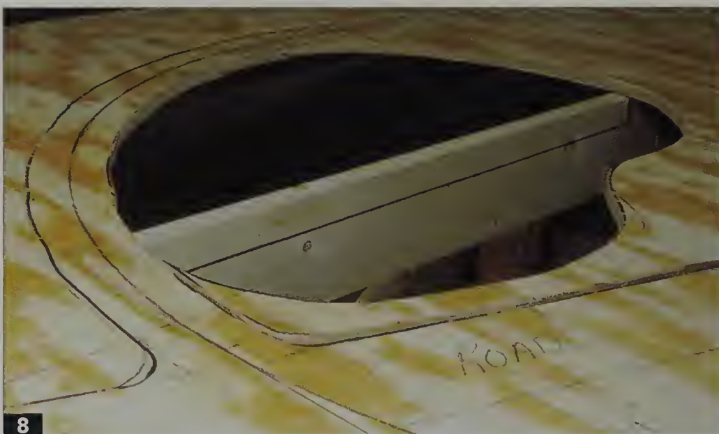
8 Dropping the lake below the table area requires cutting the joist below the lake. Here the joist has been marked.
