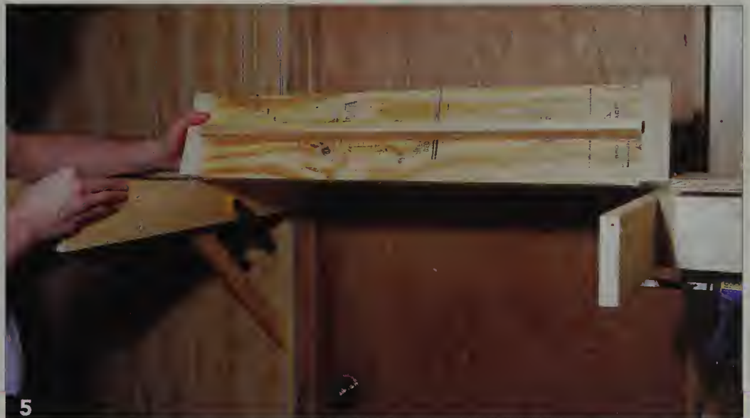
A 1 x 2 across each end provides mounting pads, and the lengthwise 1 x 2 doubles as a brace and handle.
