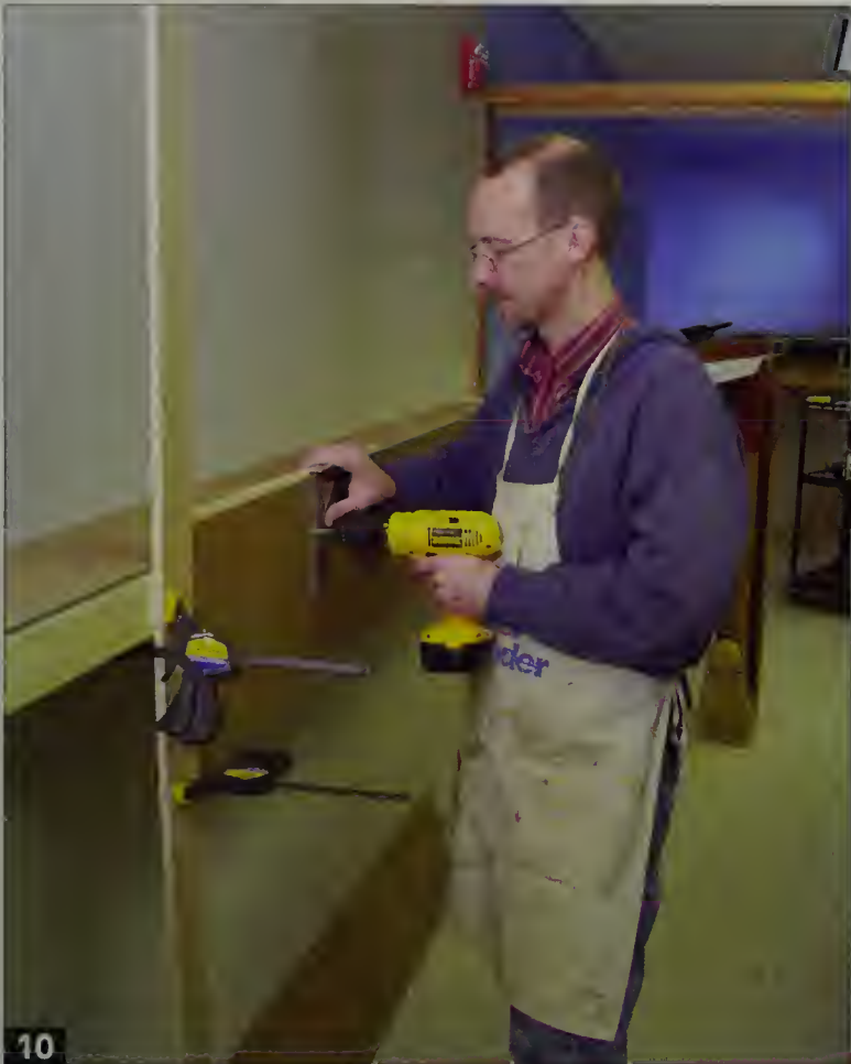
The narrow box frame takes up very little room. Fascia can be screwed to the front 1 x 3.
