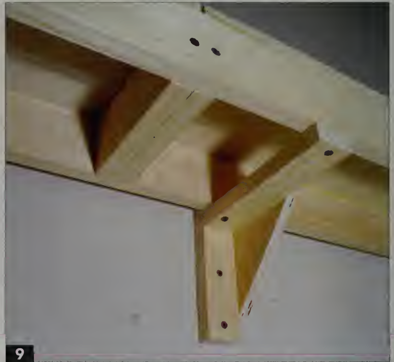
Simple homemade shelf brackets work well for narrow box-frame benchwork.
