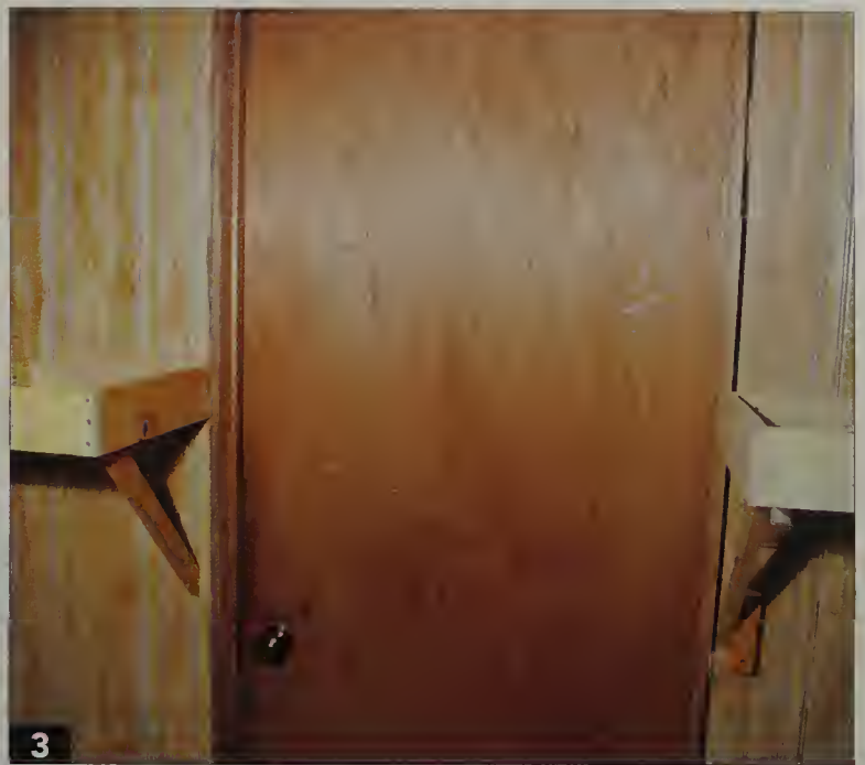
The wall-mounted, open-grid benchwork was built to either side of the doorway, with a 1 x 4 face on each side.
