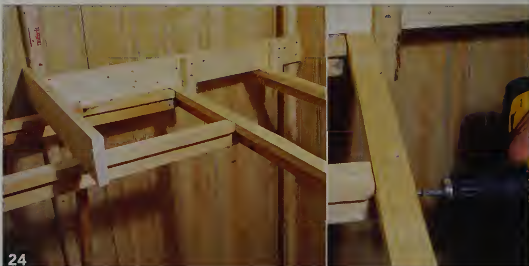
24 Cut the top flange from the two girders that are perpendicular to the original girder and then use a pair of screws to secure them.
