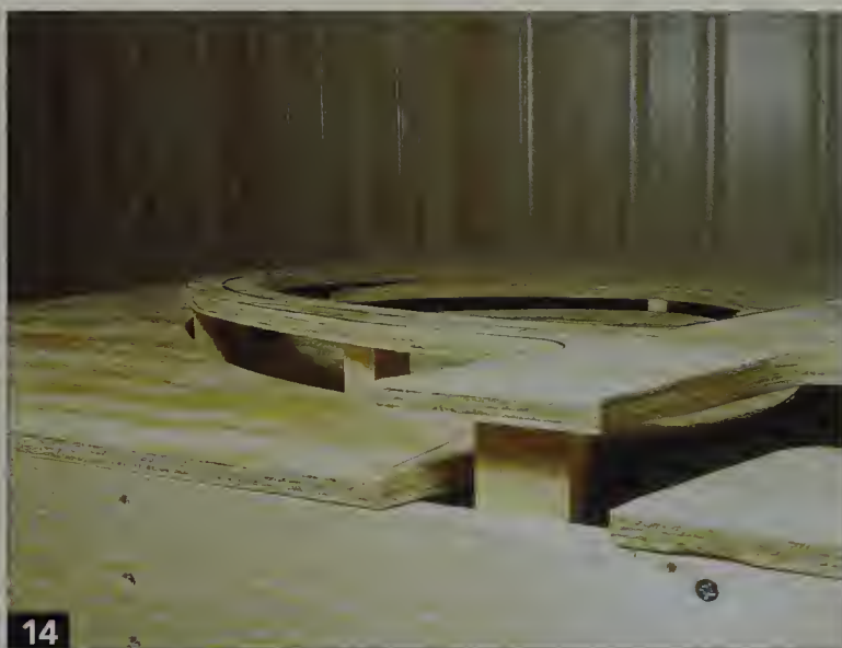
14 Clamp the intermediate risers into position, making sure the grade is smooth and even. Screw the risers into the joists.
