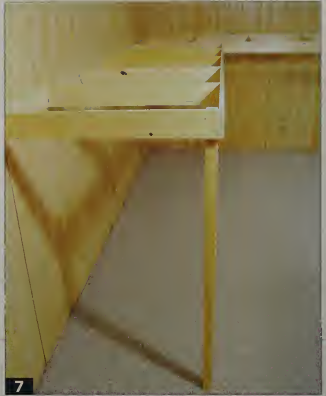
You can use standard legs with this layout style. A leg at every frame joint is usually sufficient.
