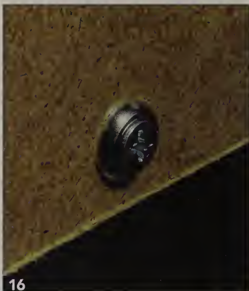
16 Wood screws with finishing washers are a good choice if you don't need a perfectly smooth finish.
