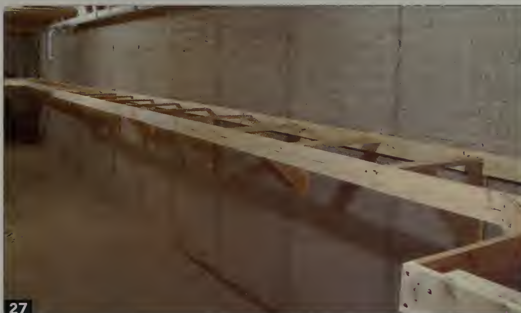
This long stretch of benchwork is anchored to a poured-concrete basement wall with a nail gun. The recessed pocket is designed to hold a 2" sheet of foam insulation board. Jim Six
