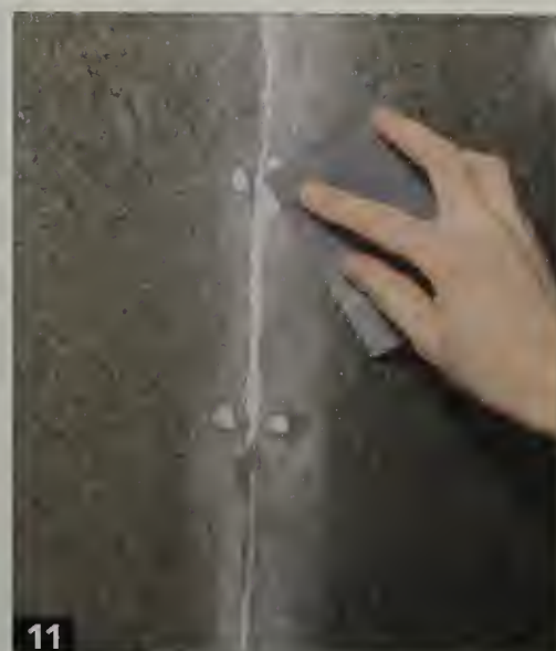
11 A fine drywall sanding sponge works well for smoothing the filler material.
