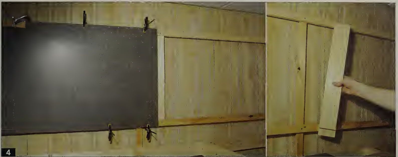
4 Clamp the first section of hardboard in place. The backing plate is a 1 x 4 that is screwed in place between the horizontal supports at the backdrop joint.
