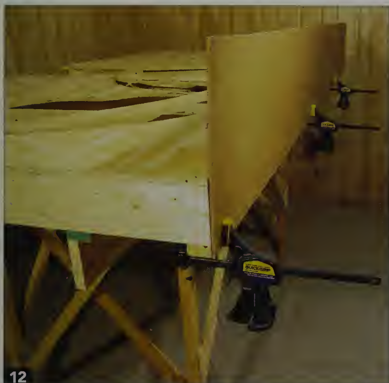
12 Clamp the hardboard fascia in place on the edge of the benchwork.
