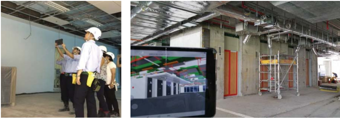
FIGURE 6-15 Viewing HVAC ducts in the BIM model on an iPad on site using the BIM 360 Glue app, during construction of the Mapletree Business Park II, Singapore. See Case Study 10-8 for more information on this project.
