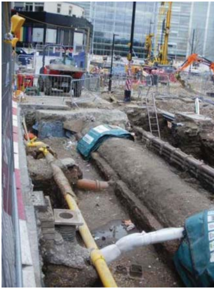
FIGURE 10–6–5 The exposed existing Victorian sewer and other buried utilities. These utilities were laser scanned and then modeled and put into the 3D model.
