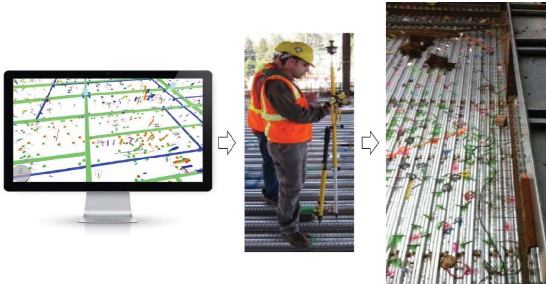
FIGURE 6-18 From model to field: layout of hangers for MEP installation in a flex deck slab shutter system prior to pouring concrete.
