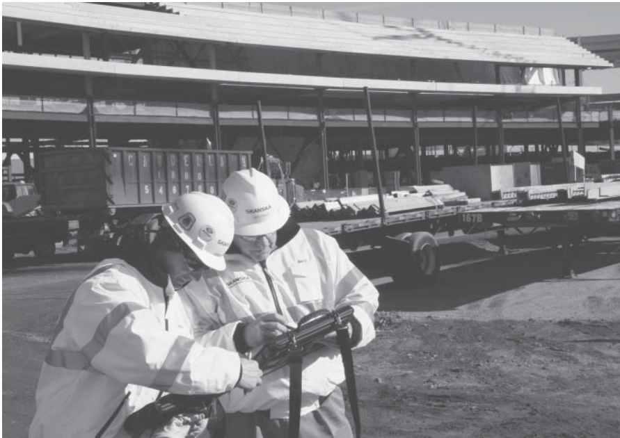
FIGURE 7-9 (Top) Field personnel use rugged tablet PCs to query information about precast pieces and their production, delivery, erection, and approval status from a color-coded model of the stadium. (Bottom) The PCs are equipped with readers to capture information from RFID tags attached to the precast concrete pieces.
