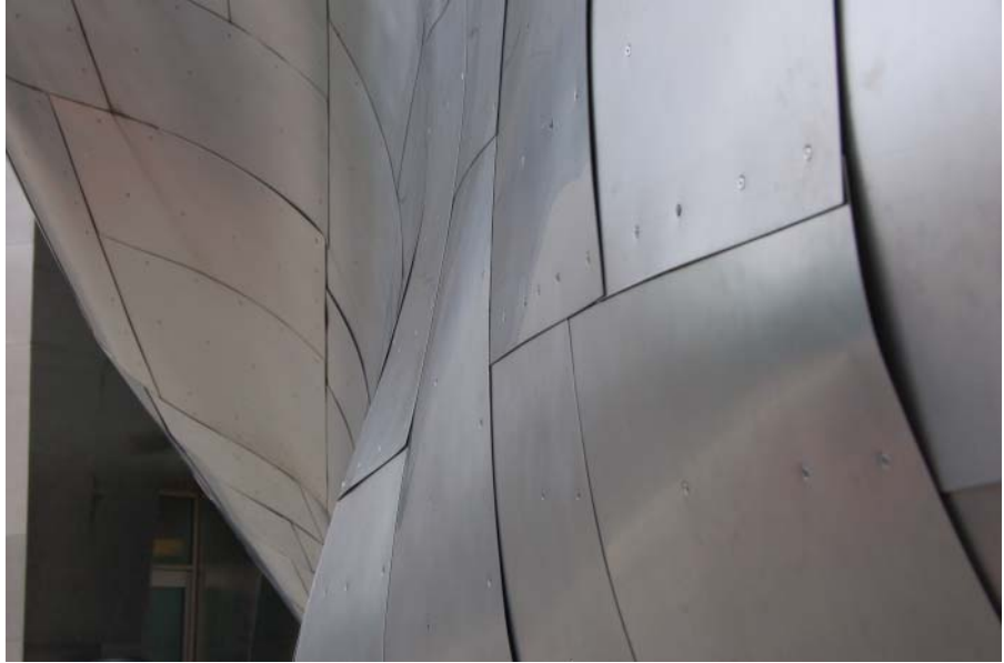
FIGURE 10-4-4 Intended gaps between panels at EMP, Seattle.
