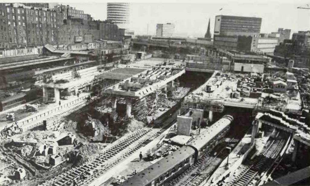
Above: The reconstruction of New Street Station, Birmingham, 1965-67.
