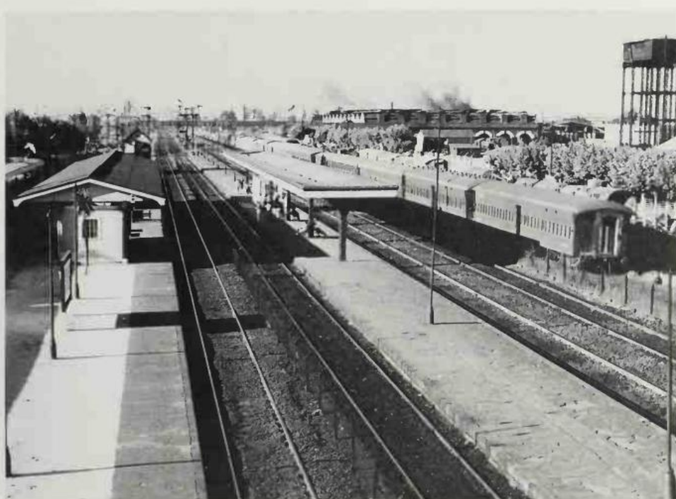
Left: Buenos Aires' suburban Escalada station, looking towards Plaza Constitucion Terminus.
