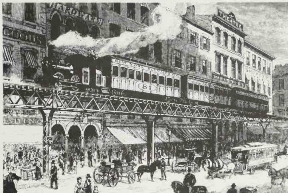
Above: New York's Third Avenue EL prior to electrification. This was, in fact, the last elevated railway to run in Manhattan proper. It closed as recently as 1950. The drawing of the locomotive (a Forney type 0-4-4T) is not totally accurate; its date is January 1879.
