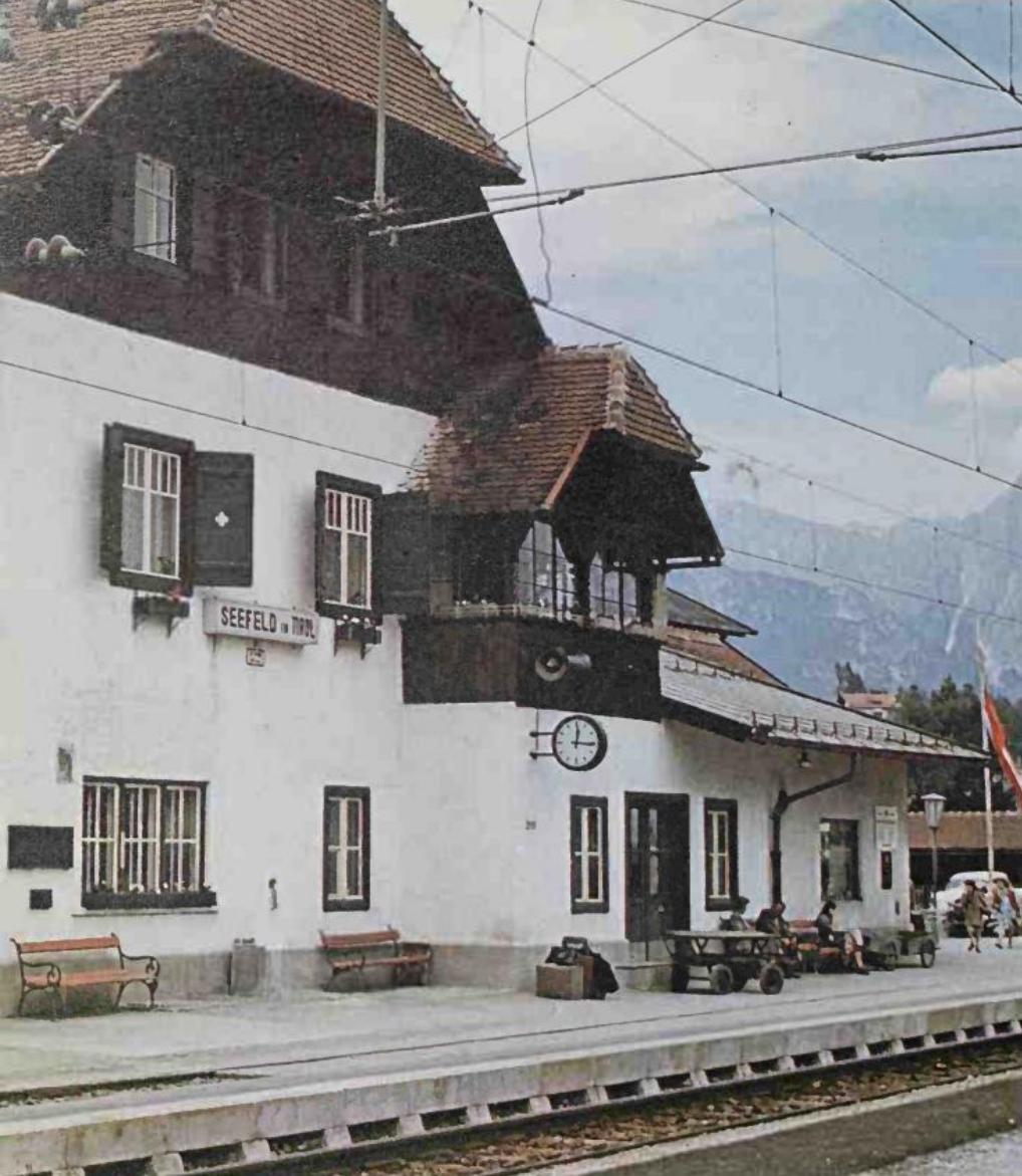
Above: A typical wayside station in the Swiss Alps.
