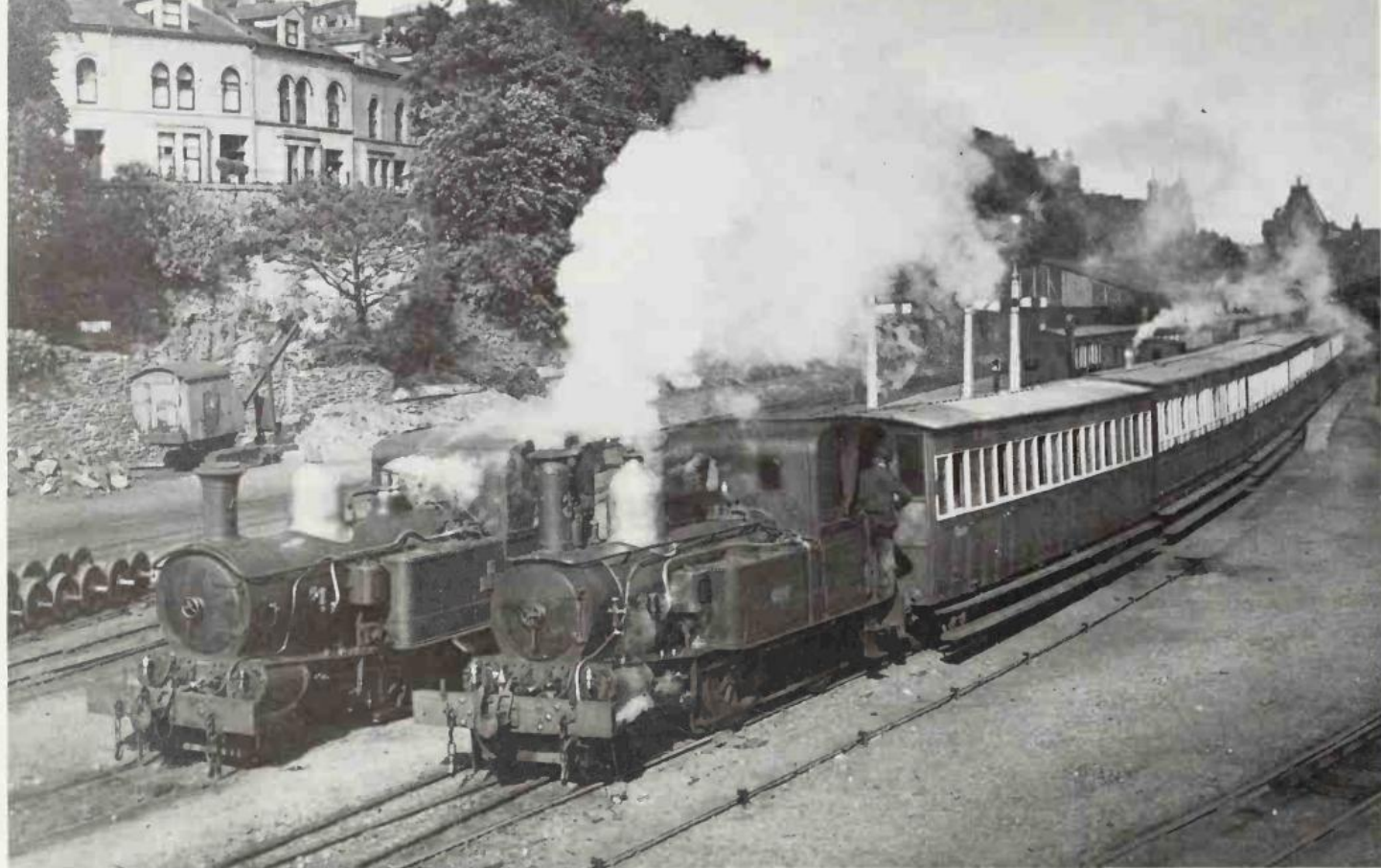
Above: Steam in the Isle of Man. Now a government-sponsored tourist line and using only a truncated section of its original network (Douglas-Port Erin) this 3ft 6in gauge railway has always been unique. Its locomotives, all 2-4-0 tank engines (bar one), were built by Beyer Peacock of Manchester and a typical example of that firm's Victoriana; its coaches were equally ancient. Today these museum pieces travel the tracks during the summer as part of the Island's holiday attractions. This photograph was taken in 1956 and shows the terminal station at Douglas when trains ran to Port Erin, Peel and by the circuitous route to Ramsey.
