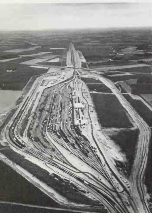
Above: Along with other major US railroads, the Norfolk & Western constructed its own electronically controlled classification yards. Pictured above are the facilities at Bellevue, Ohio in 1967.
