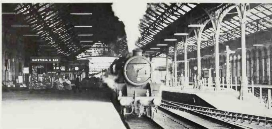
Above: Preston, on the west-coast line from London to Scotland appears much the same in this 1965 photo as it was in the Edwardian era.
