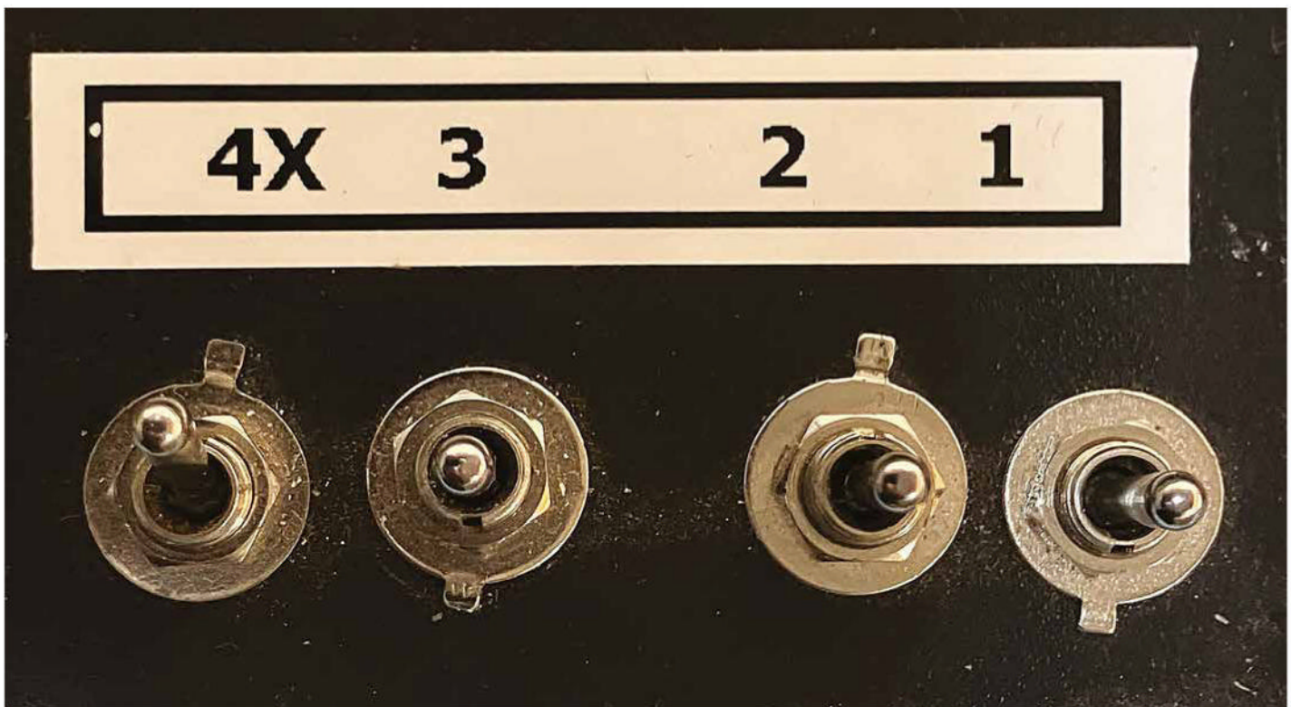
Photo 5. A small panel of DPDT toggle switches is used to operate the slow-motion point motors in the goods train section of the staging yard; these are marked with a red dot on Figure 1. It is possible to operate both points that form a crossover with the one switch. The wiring to one motor needs to be the opposite way around to the other set used to form the crossover.
