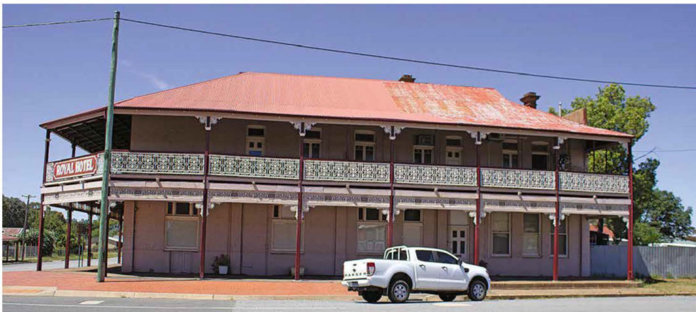
The majestic Royal Hotel. Modelling the roof in the process of being repainted might make an interesting modelling detail.
