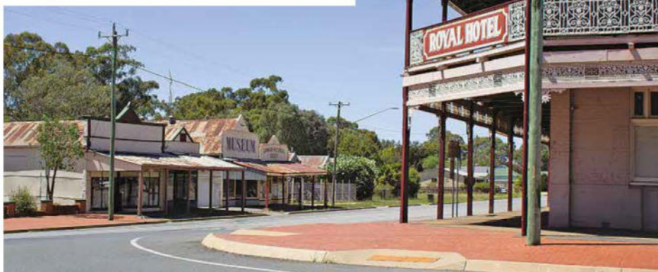
► The junction of Ford St and Waterview St shows this very traditional street scene. Note the different verandah heights and the centre sinking on the Museum. It's worth contemplating adding some of these odd features to your layout.
