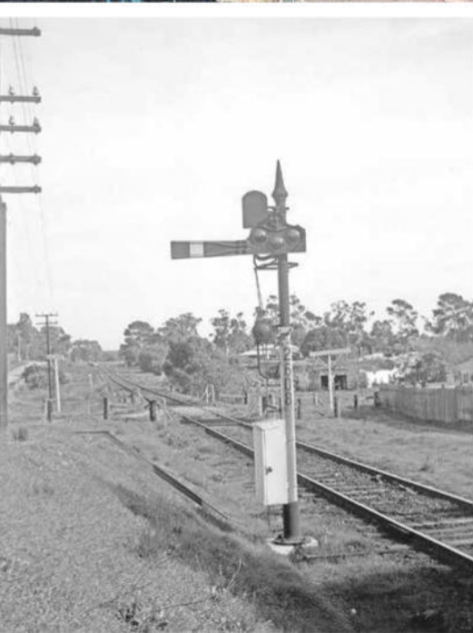
◀ Photo 10. This 1952 image shows the short upper quadrant signal No. 2608 positioned at the up side of the King Street bridge. The reduced height of this signal enables drivers to sight the aspect through the King Street bridge.
