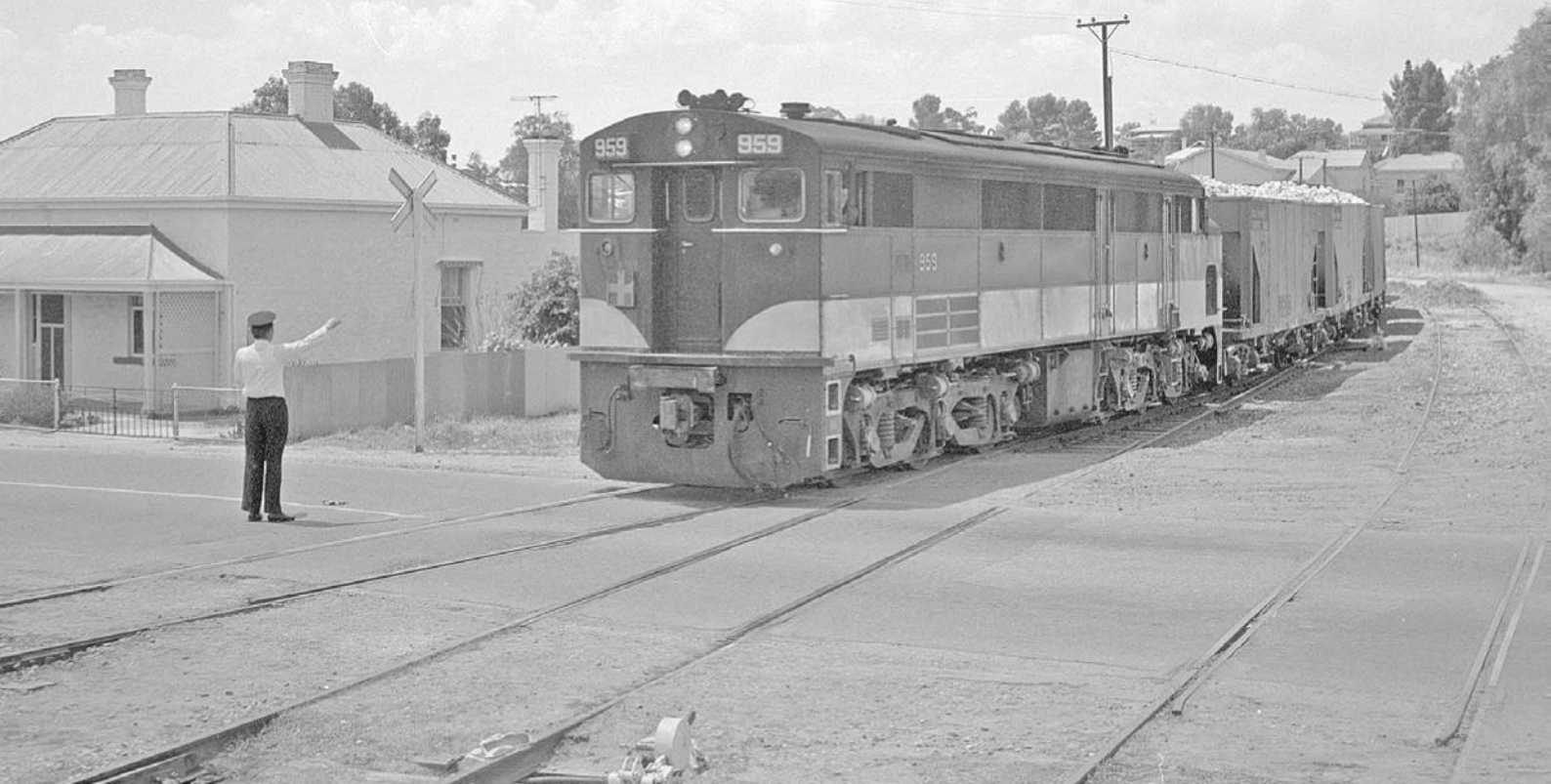
Photo 8. In this 1972 image the Penrice Stone train is being hauled by locomotive No. 959 into North Gawler and is crossing Murray Street. The station master is holding a stop board and is about to collect the staff from the crew.
