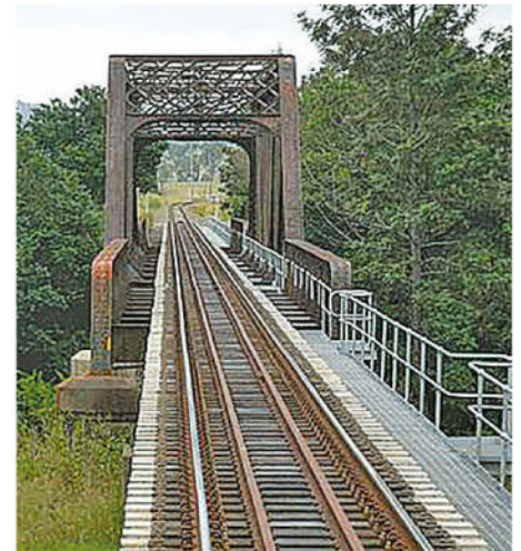
▲ Photo 12. The prototype Williams River bridge photo by James Brook.
