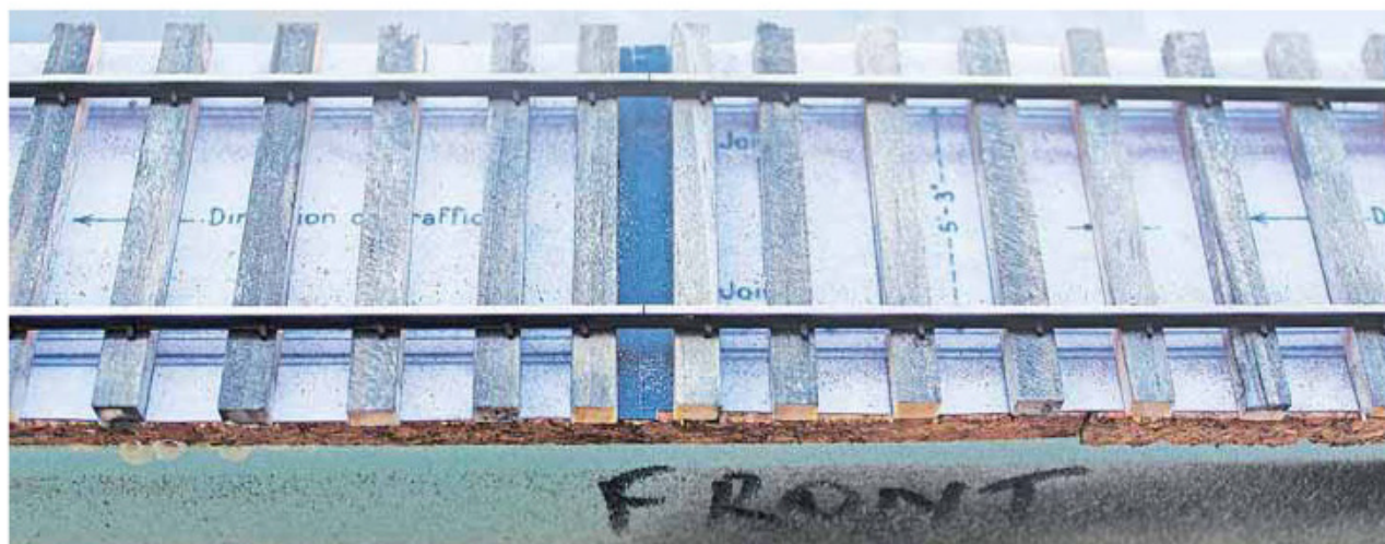
Once the first rail has been secured, the second rail is gauged to the first rail with the help of Fast Tracks sweep sticks. I usually spike about 300mm (less on curves) on one side before removing the sweep stick and securing the other rail. Then the gauge is checked against a NMRA standards gauge and adjusted if necessary. To finish, notches will be cut in the rail head to simulate joints and cosmetic fishplates will be soldered to the rail. The rails will then be painted.
