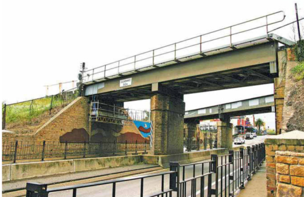
The dual road overbridge at north-western end of the rail yard at Muswellbrook in 2016. Photo Trevor Hodges.
