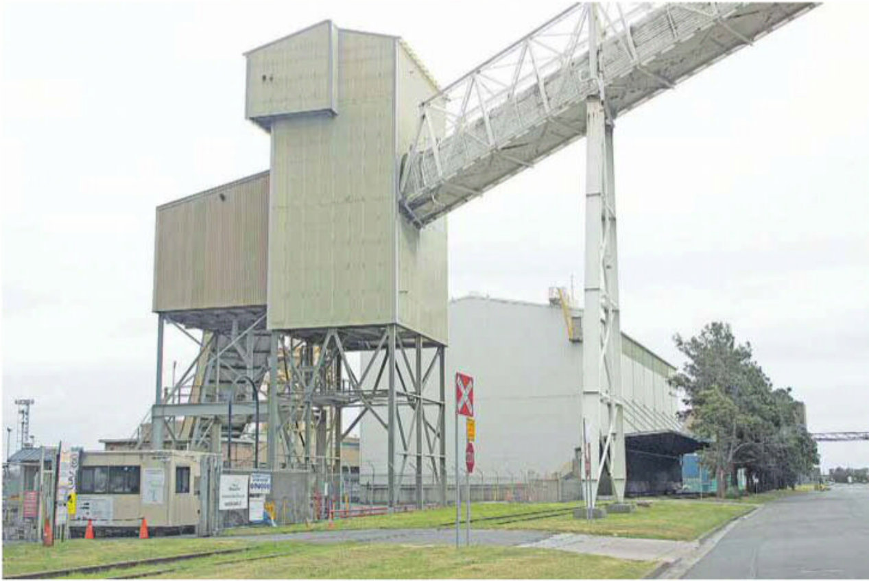
7 Looking north and situated just south of the Cargill facility, is this conveyer which straddles Heron Road. Industrial structures such as this look like they are straight from a 'Walthers' catalogue. Improvisation and kit bashing can produce good results. Note the signage on the level crossing.
