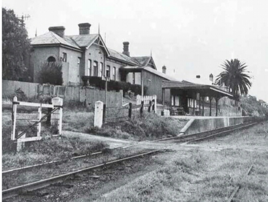
Another photo of the third and final Morpeth station and platform, this time taken from the down side looking up the line heading out of town toward East Maitland. The Robert Street level crossing is visible in the foreground.
