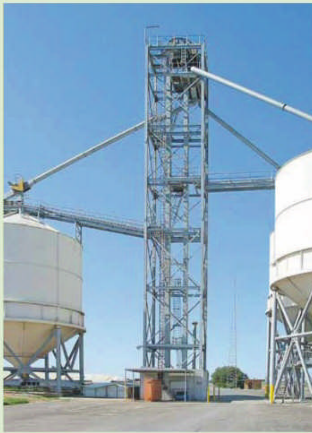
This is the distribution tower that sits between the two dumper bins and the four auxiliary bins. To the left of the tower is a bottom dump facility for road vehicles, enabling quick additional top-ups to the bins.
