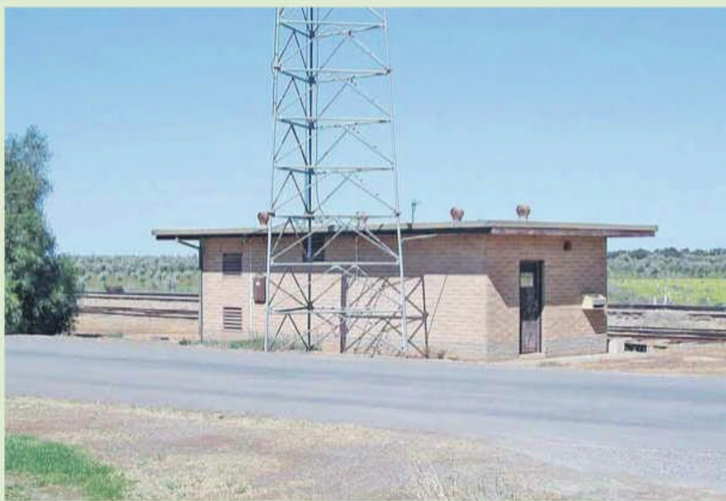
One of the few 'railway' buildings at Bowmans: the relay cabin.
