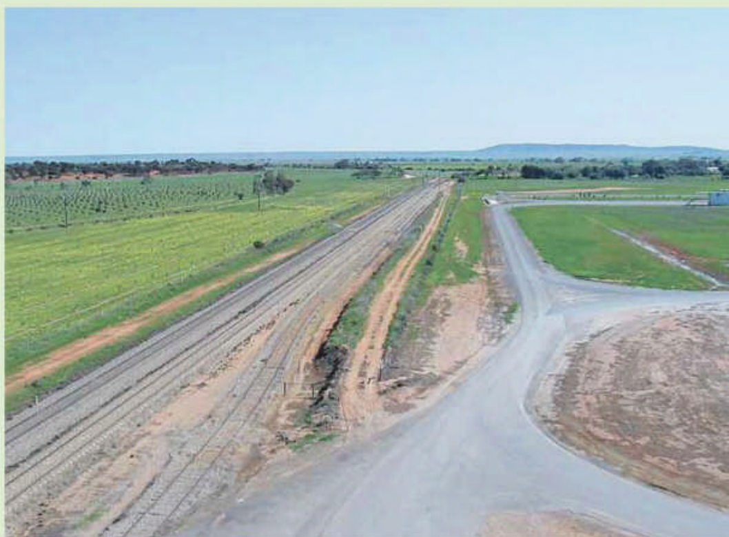
Looking north. The main line is on the left, then the crossing loop; the third track is the dead-end siding fed by the grain bins. The roads within the facility are all-weather asphalt roads.
