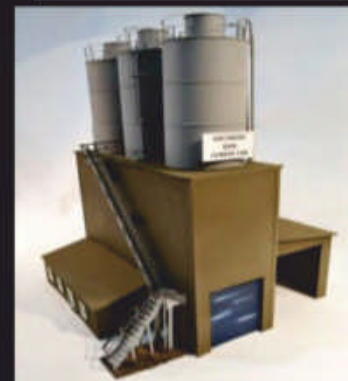
TS5 - CEMENT WORKS
