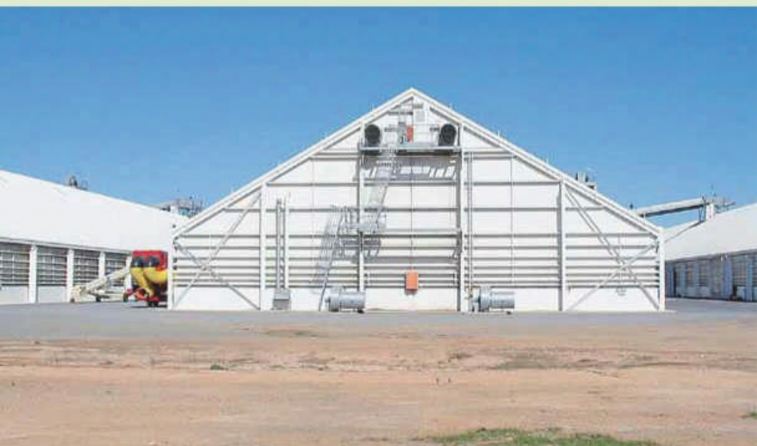
The northern end of the permanent bunkers.
