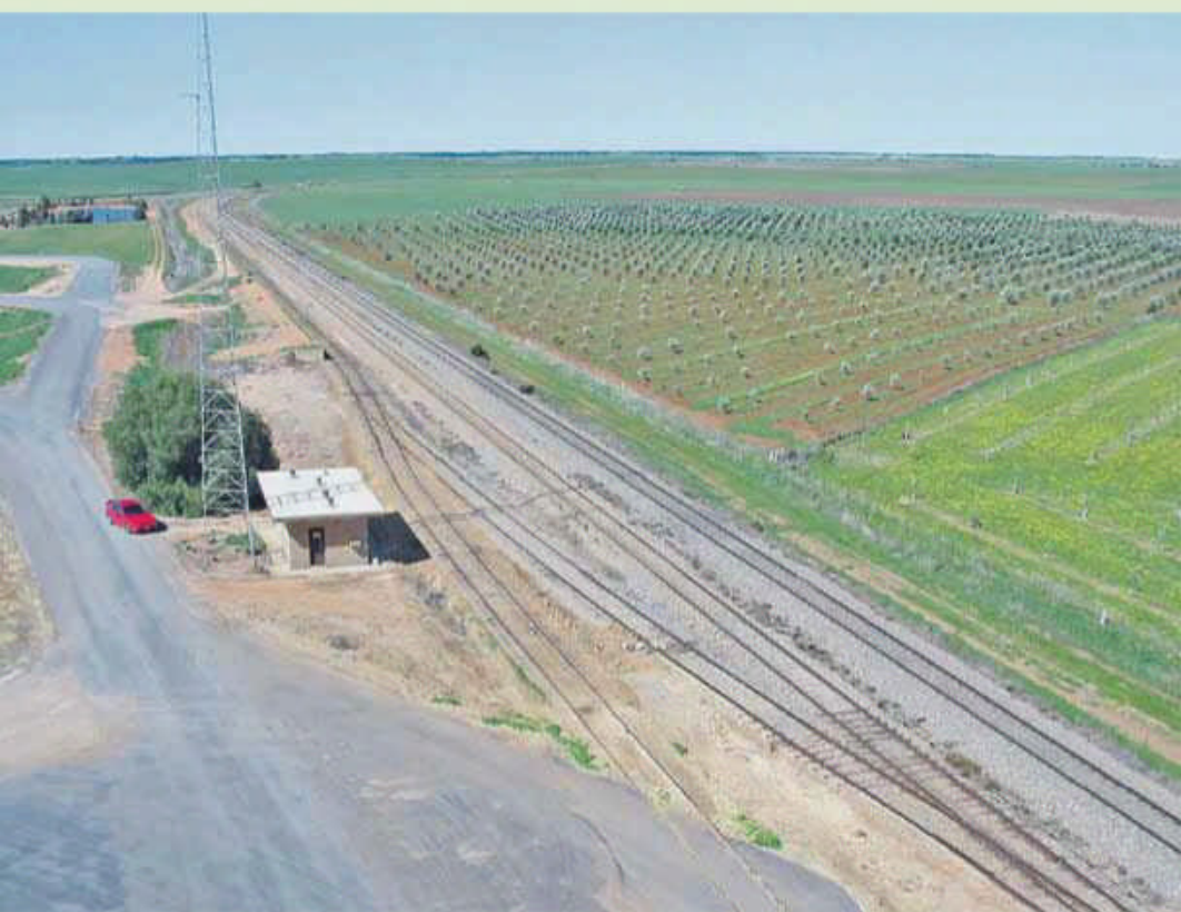
Looking south. To the right is the main line, then the crossing loop, with the crossover to the goods loop. Between these two points you can see the derail. The siding closest to the relay cabin is fed by the grain bins. The repeater tower can be seen behind the relay cabin. The goods platform has been used in the past to 'top up' grain trains while loading, using portable augers.
