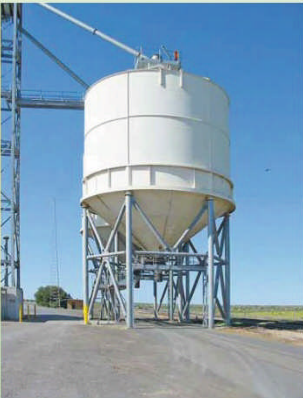
The grain bins. There are two outlets for loading and steps for staff to accomplish and supervise the loading operation from a mezzanine level. The track is sunk in asphalt so road trucks can be loaded using the same bins if required.
