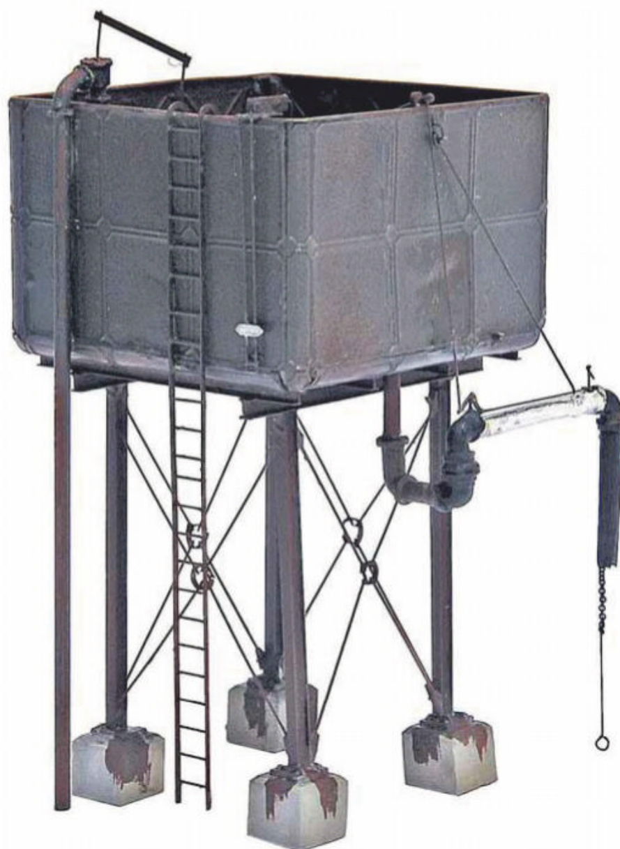
The 10,000 gallon tank, showing details of the water crane jib and other external fittings.
