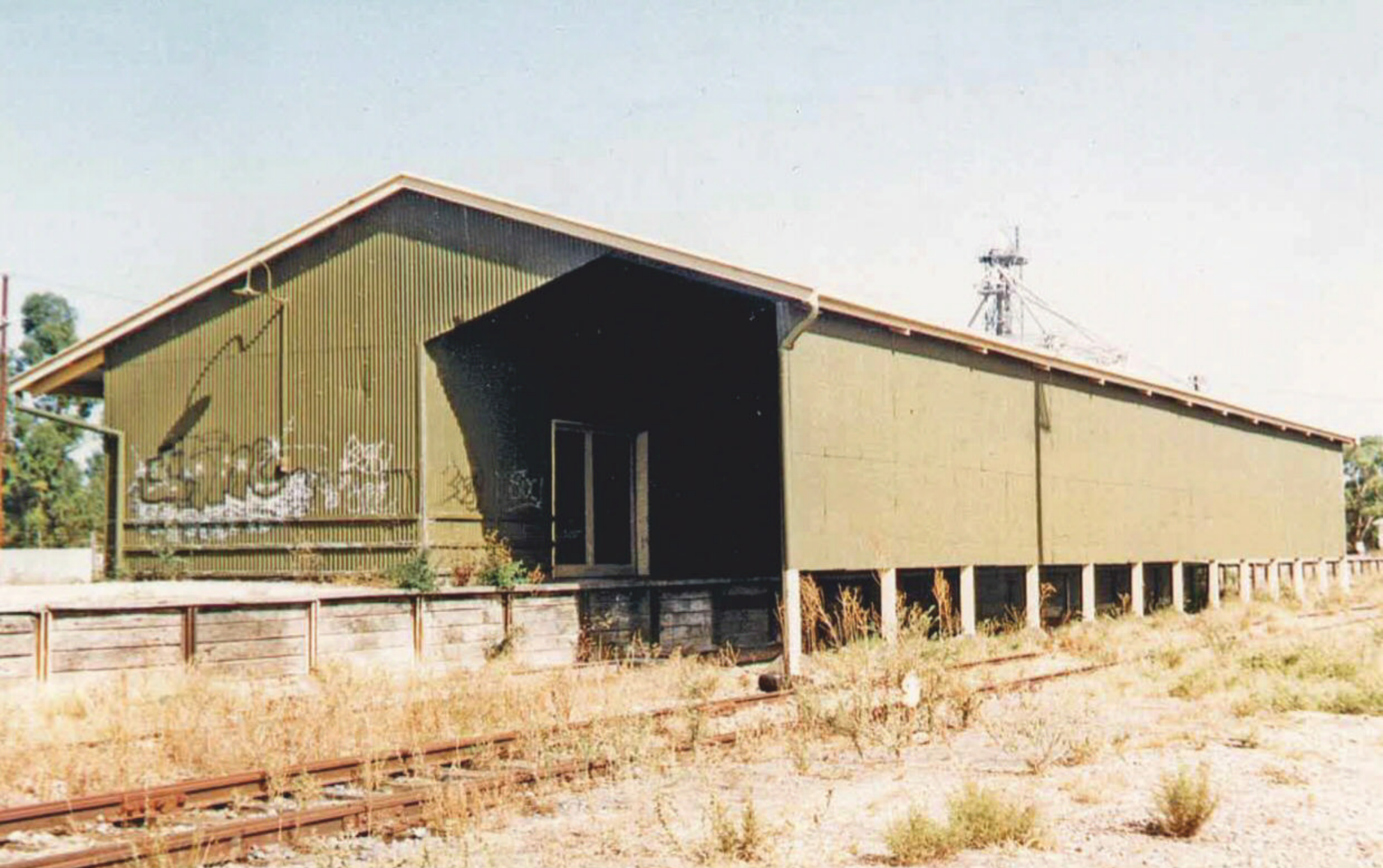
The gable-roofed, corrugated iron-clad goods shed at Naracoorte in the south east of South Australia. In subsequent articles in this series, the author will show how he constructed a shorter version of this design of SAR goods shed in HO scale. Photo by Gavin Thrum.
