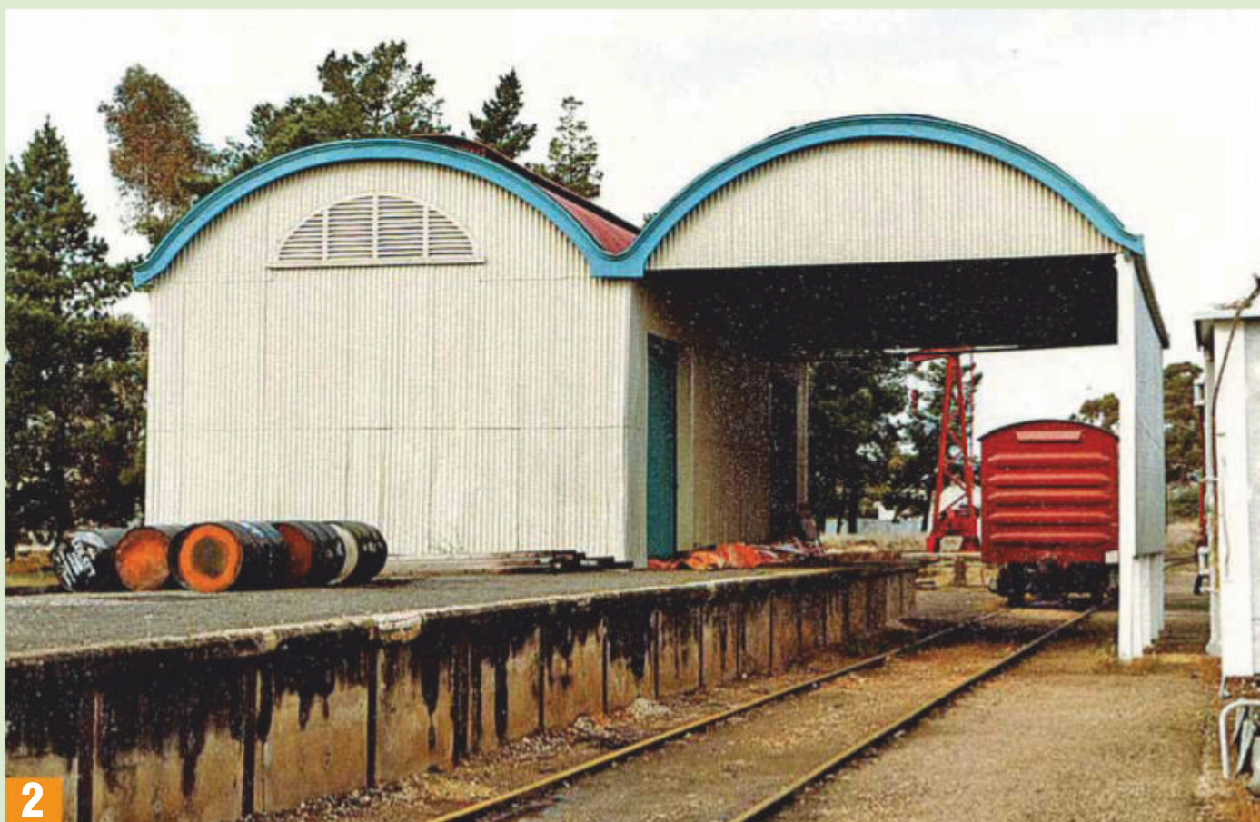
2 The double barrel roof design, illustrated by the now demolished goods shed at Nuriootpa, photographed in 1981.
