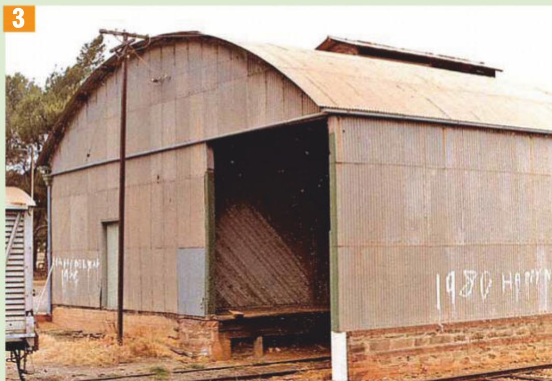
3 The barrel roofed goods shed at Tarlee, complete with large roof vent and dwarf stone wall holding up the rail-side timber-framed corrugated iron-clad wall.
