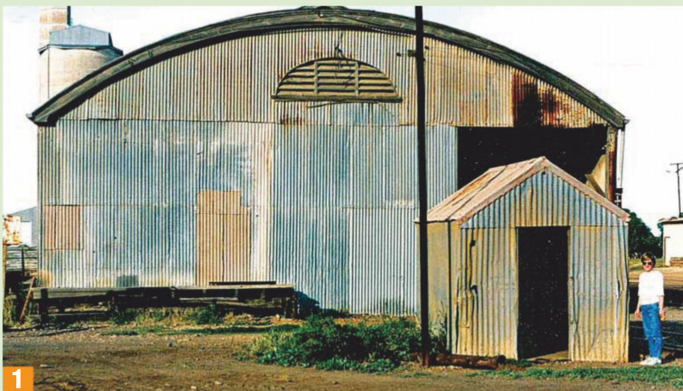
1 The round (barrel) roof iron-clad goods shed at Quorn.
