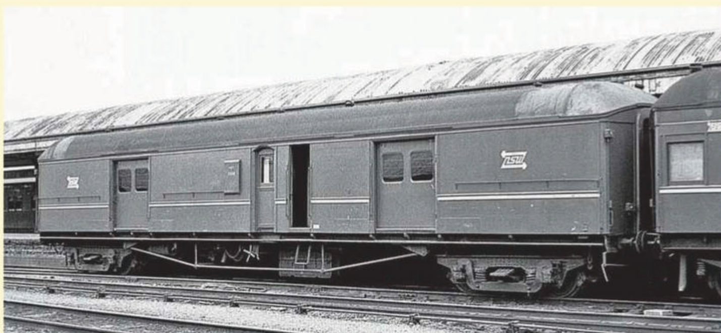
Showing its final form as a VHO with plain side sheeting with no letterboard, as well as the second type of modified guard's compartment, VHO2650, one of the Clyde Engineering-built vehicles delivered in 1928, stands at one of the Sydney Terminal platforms. The image was captured some time between September 1974, when it was renumbered from 1805, and December 1980, when it was rebuilt as an MHO. Photo from the Ian Dunn collection.
