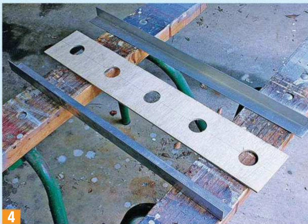
4 A crossbeam for Morpeth under construction. Two pieces of aluminium angle cut to length, 'sandwiching' a 3mm ply spacer which has had five 25mm holes drilled along its length, to lighten the timber and allow a convenient route for the of wiring along the baseboard.
