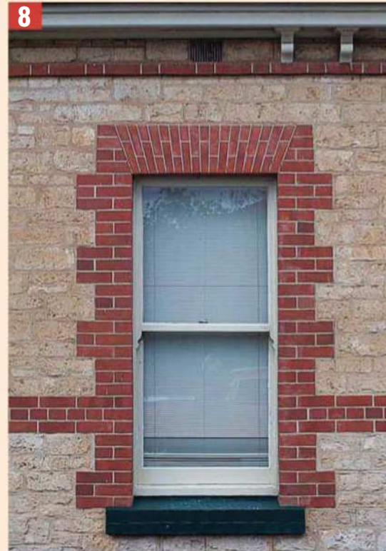
A slightly different arrangement of the brick quoining around another window of a community centre building in the southern suburbs of Adelaide.
