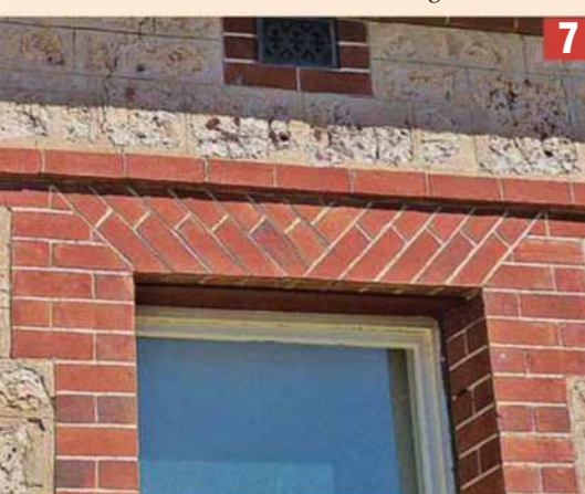
▼ Detail of the brickwork around the windows and the ventilator above on a community centre building in the southern suburbs of Adelaide. It is typical of the window and vent treatments of the era during which the Booleroo Centre station building was built.
