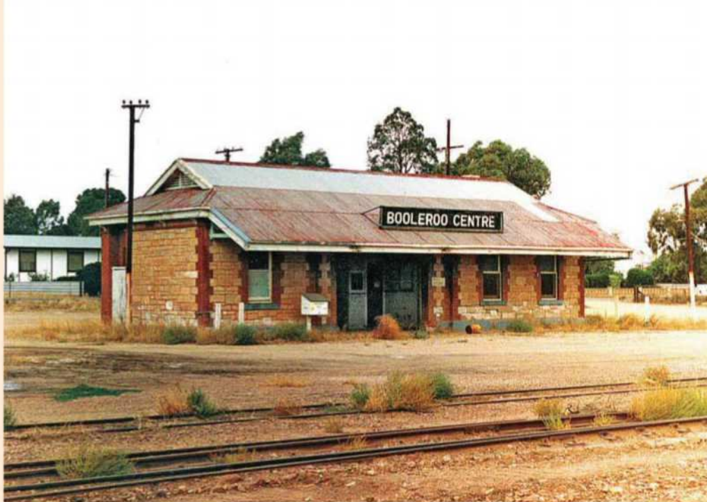
The rail side of the dressed stone building at Booleroo Centre, photographed during the late 1980s.
