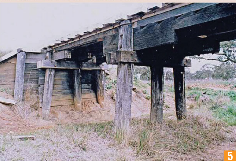
Detail of the piers, wing walls and girders of the bridge near Towealgra.
