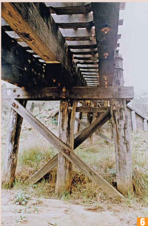
Detail of a pier and the underside of the girders and transoms of the bridge near Towealgra.
