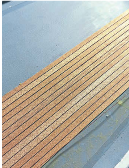
Planking the deck, using string between the planks for better definition.
