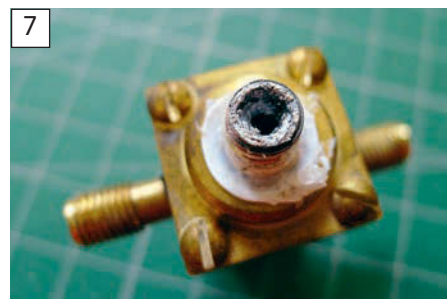
A sound reason for not keeping a valve directly attached to the boiler shell is the fact that scale and sludge can build up inside the valve steam space. While Richard's old valve was still working when last used, he knew it was only a matter of time before it seized up.
