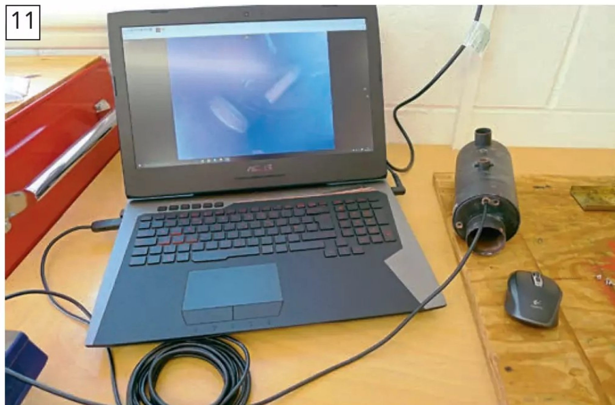
The picture isn't perfect but good enough to see the silver soldered joints and the general condition and cleanliness of the internal surfaces.
