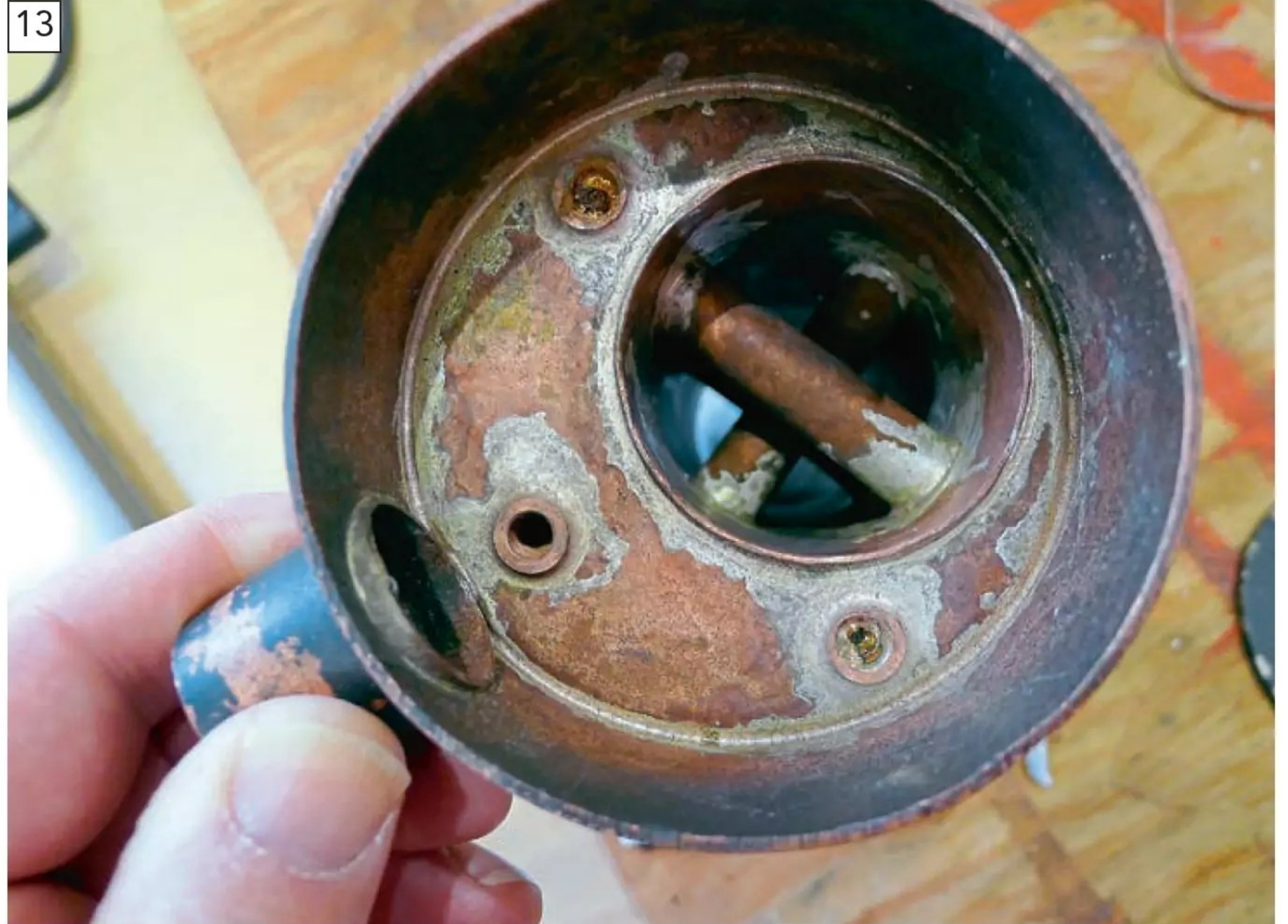
With the ends removed and a clean flat surface remaining, the boiler could be sent away to the repair shop to have the new bushes silver soldered to the ends of the tie rods.
